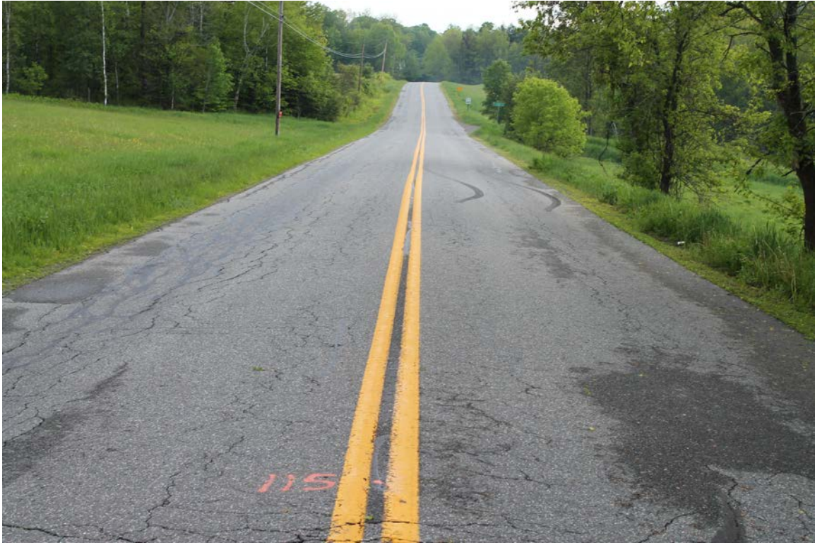
Howe Hill Road: Photo taken 5/31/2017 at station 115+00.
