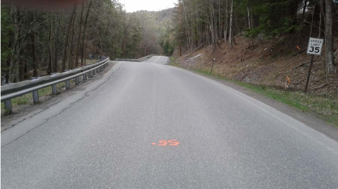
Rte #132: Photo taken 5/3/2017 at station 55+00.
