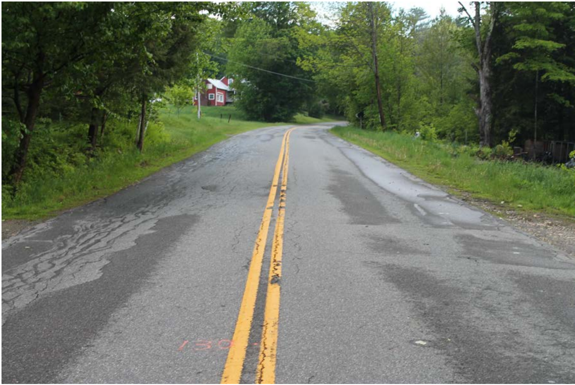
Howe Hill Road: Photo taken 5/31/2017 at station 130+00.
