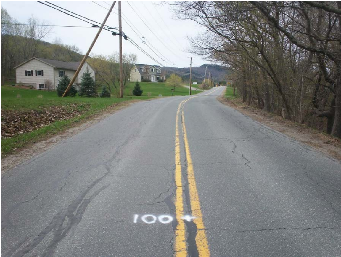
River Road: Photo taken 2015 at station 100+00 (before shim, overlay, chip seal).
