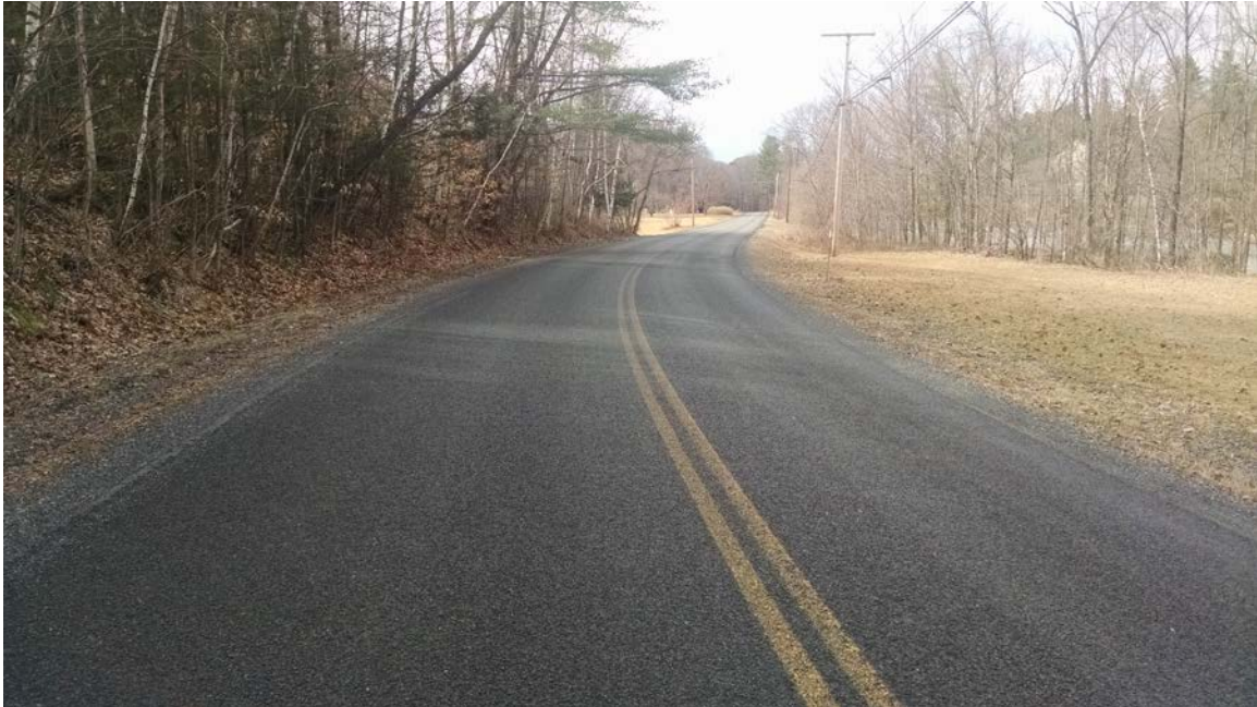
River Road: Photo taken 2015 of the final 10% rubber chip seal.
