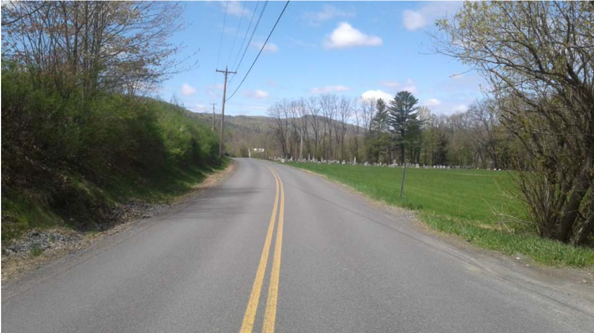
River Road: Photo taken 5/11/2017 at station 70+00.
