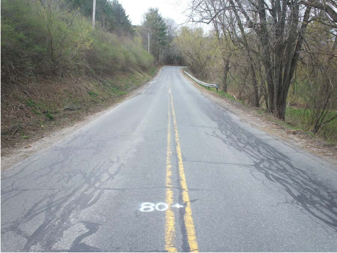
River Road: Photo taken 2015 at station 80+00 (before shim, overlay, chip seal).
