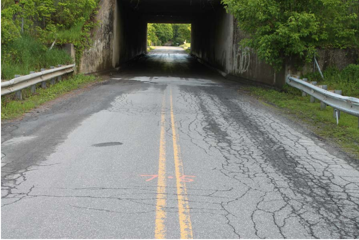
Broad Brook Road: Photo taken 5/31/2017 at station 7+50.
