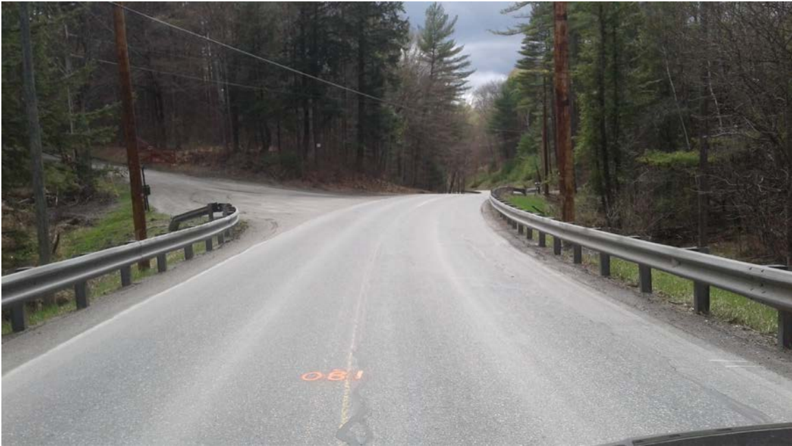
Rte #132: Photo taken 5/3/2017 at station 180+00.
