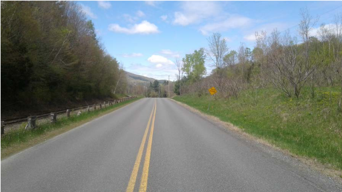
River Road: Photo taken 5/11/2017 at station 60+00.
