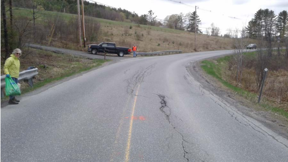
Rte #132: Photo taken 5/3/2017 at station 85+00.
