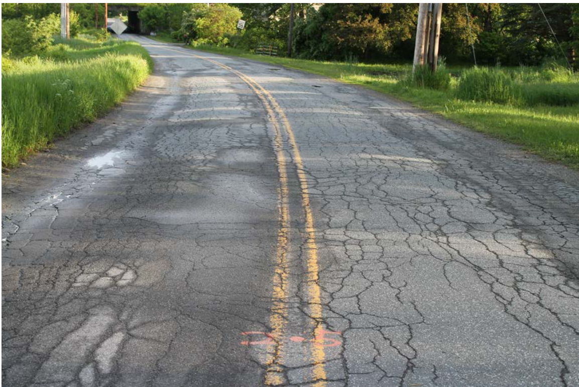
Broad Brook Road: Photo taken 5/31/2017 at station 2+50.
