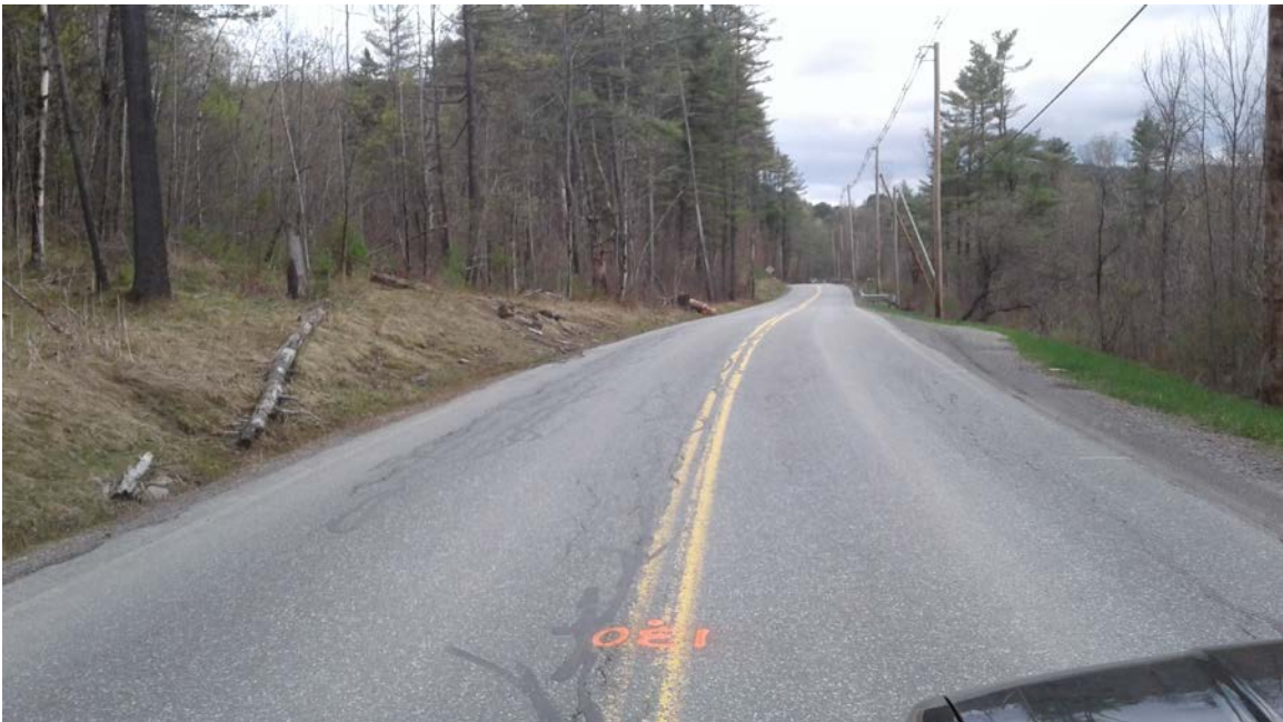
Rte #132: Photo taken 5/3/2017 at station 130+00.
