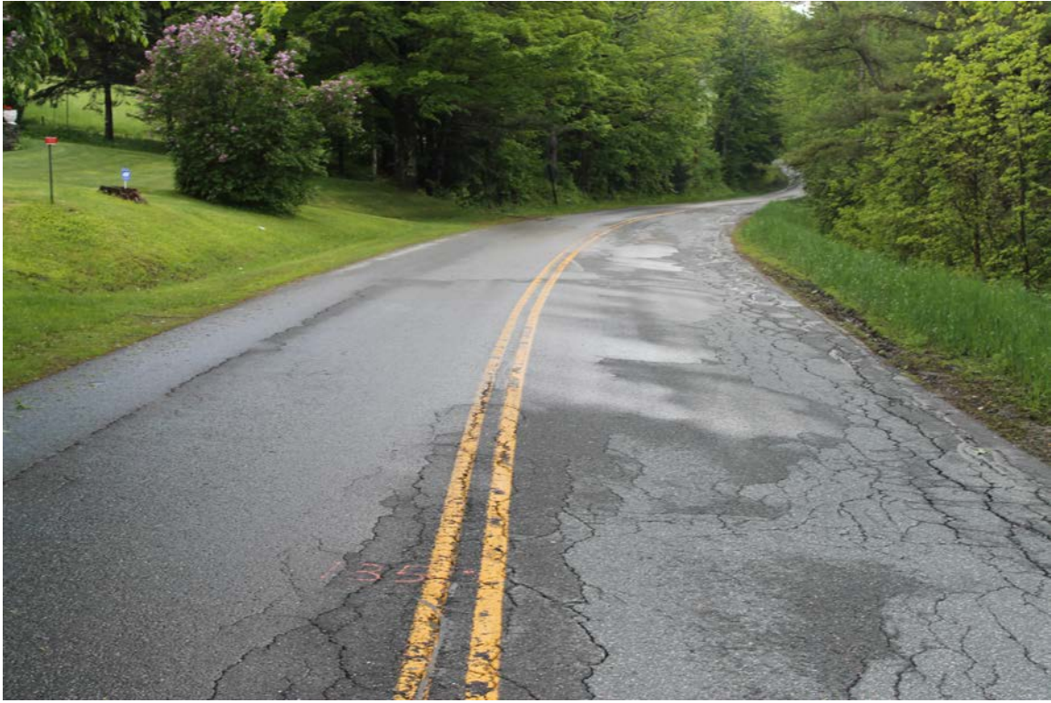
Howe Hill Road: Photo taken 5/31/2017 at station 135+00.
