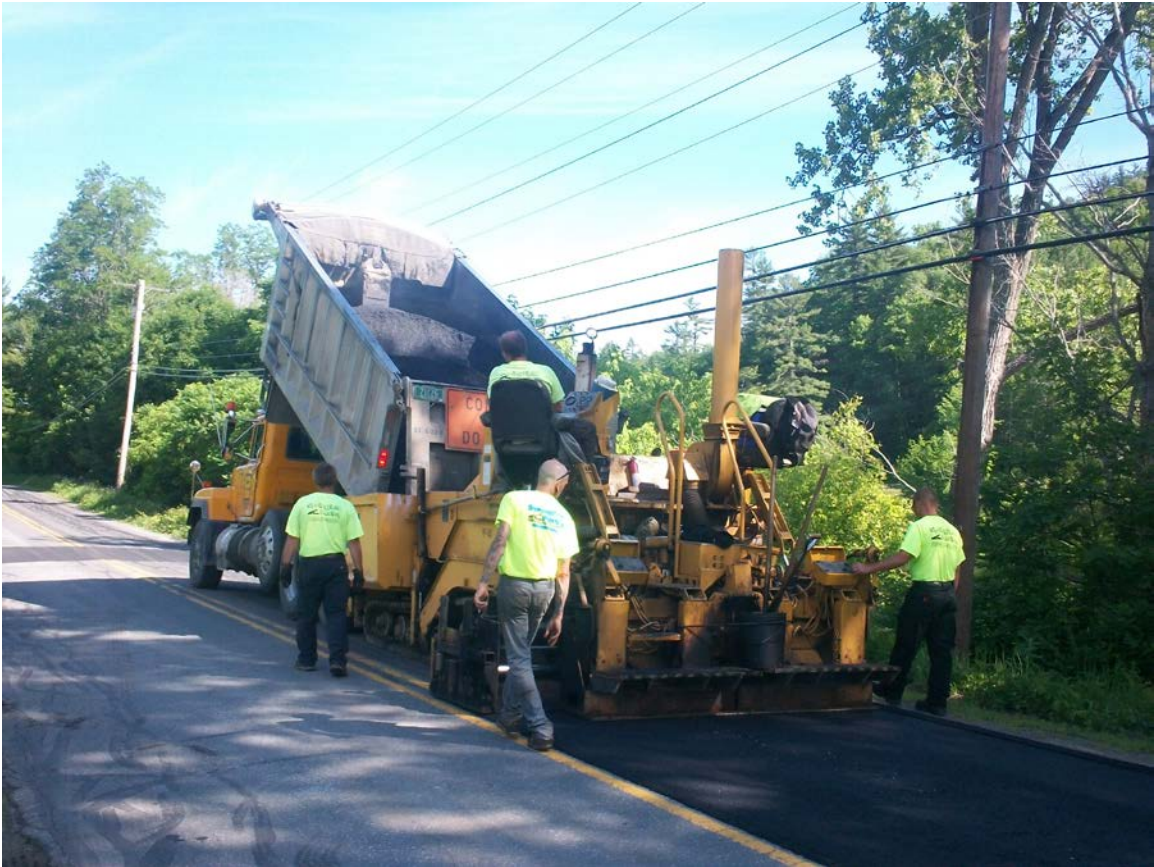
River Road: Photo taken 2015 during an asphalt shim (Station 33+00 to 126+10).
