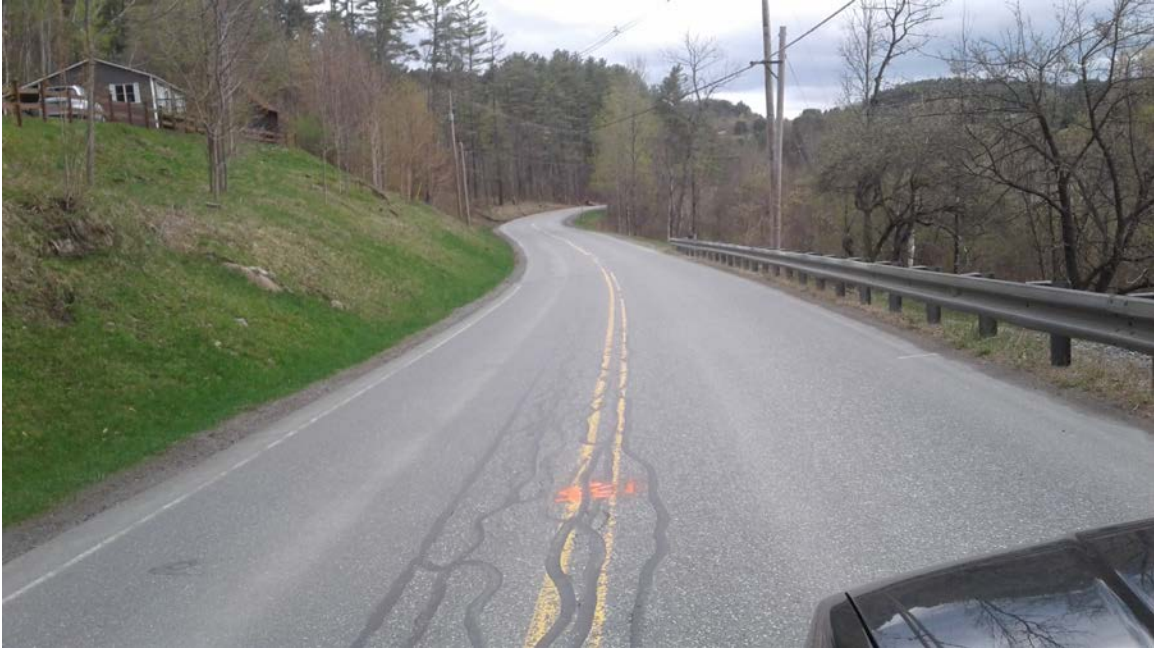
Rte #132: Photo taken 5/3/2017 at station 135+00.
