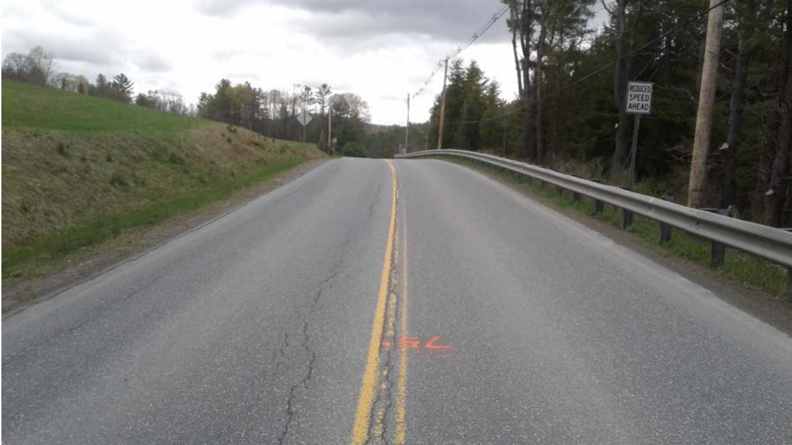
Rte #132: Photo taken 5/3/2017 at station 75+00.
