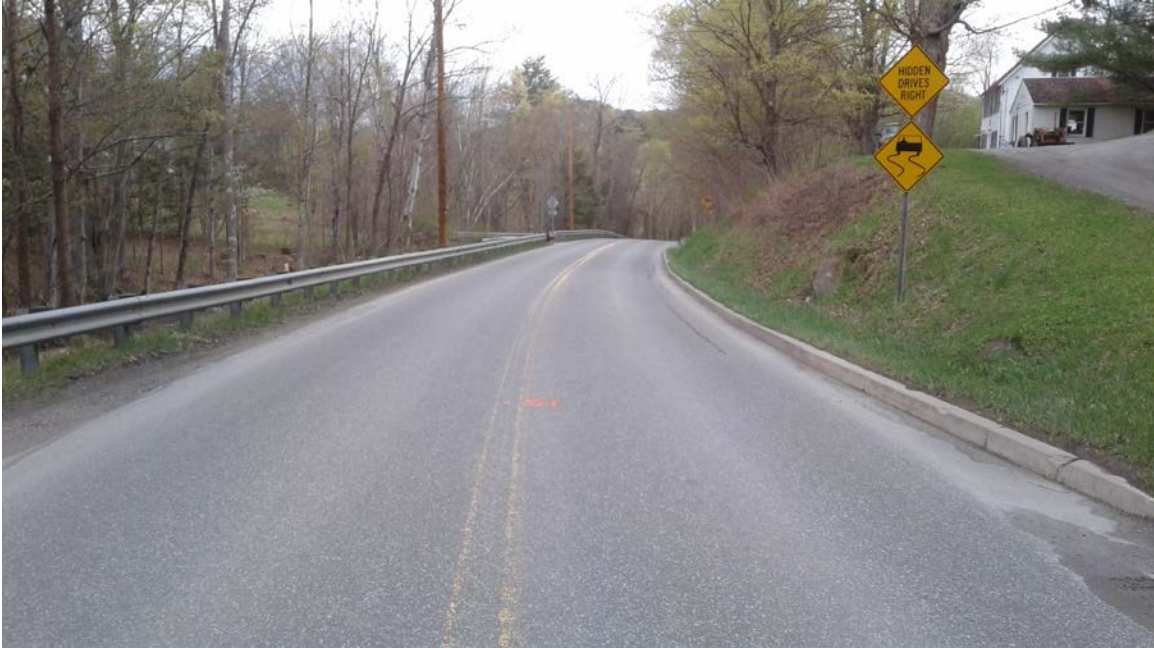
Rte #132: Photo taken 5/3/2017 at station 15+00.
