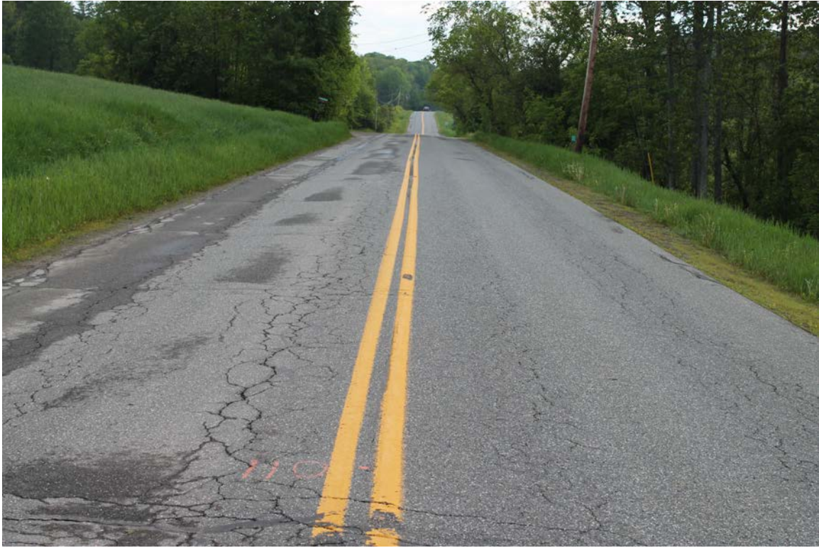
Howe Hill Road: Photo taken 5/31/2017 at station 110+00.
