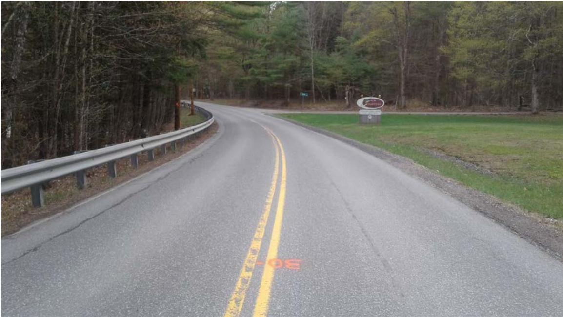
Rte #132: Photo taken 5/3/2017 at station 30+00.
