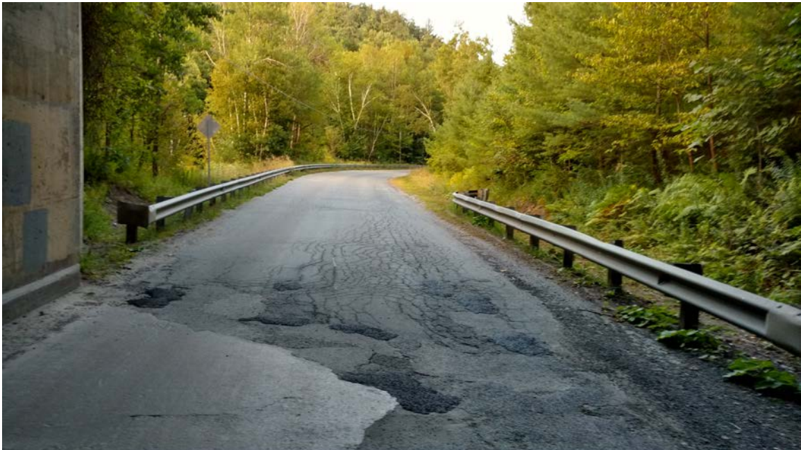
Quimby Mountain Road: Photo taken 8/31/2017 at station 14+00.
