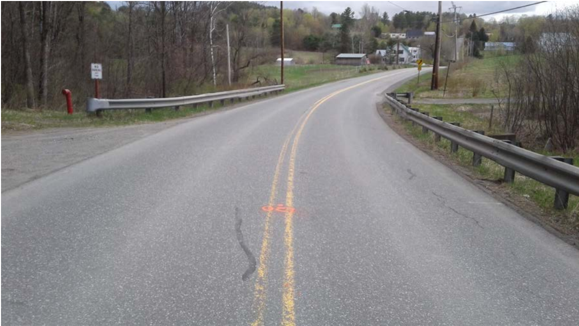
Rte #132: Photo taken 5/3/2017 at station 120+00.
