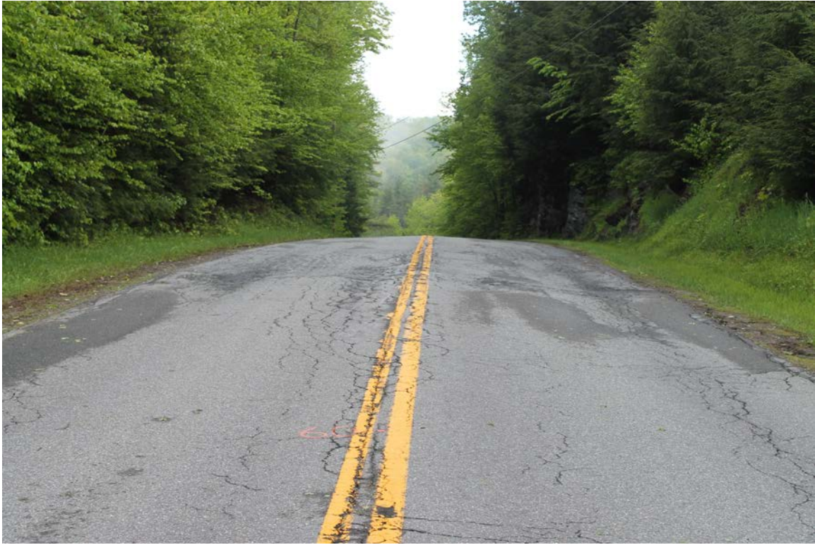
Howe Hill Road: Photo taken 5/31/2017 at station 60+00.
