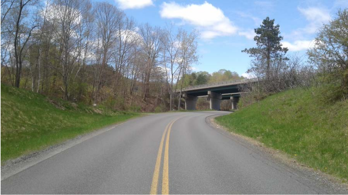
River Road: Photo taken 5/11/2017 at station 50+00.
