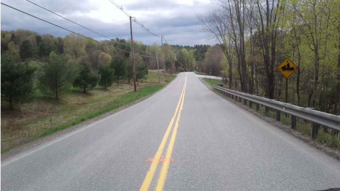
Rte #132: Photo taken 5/3/2017 at station 195+00.
