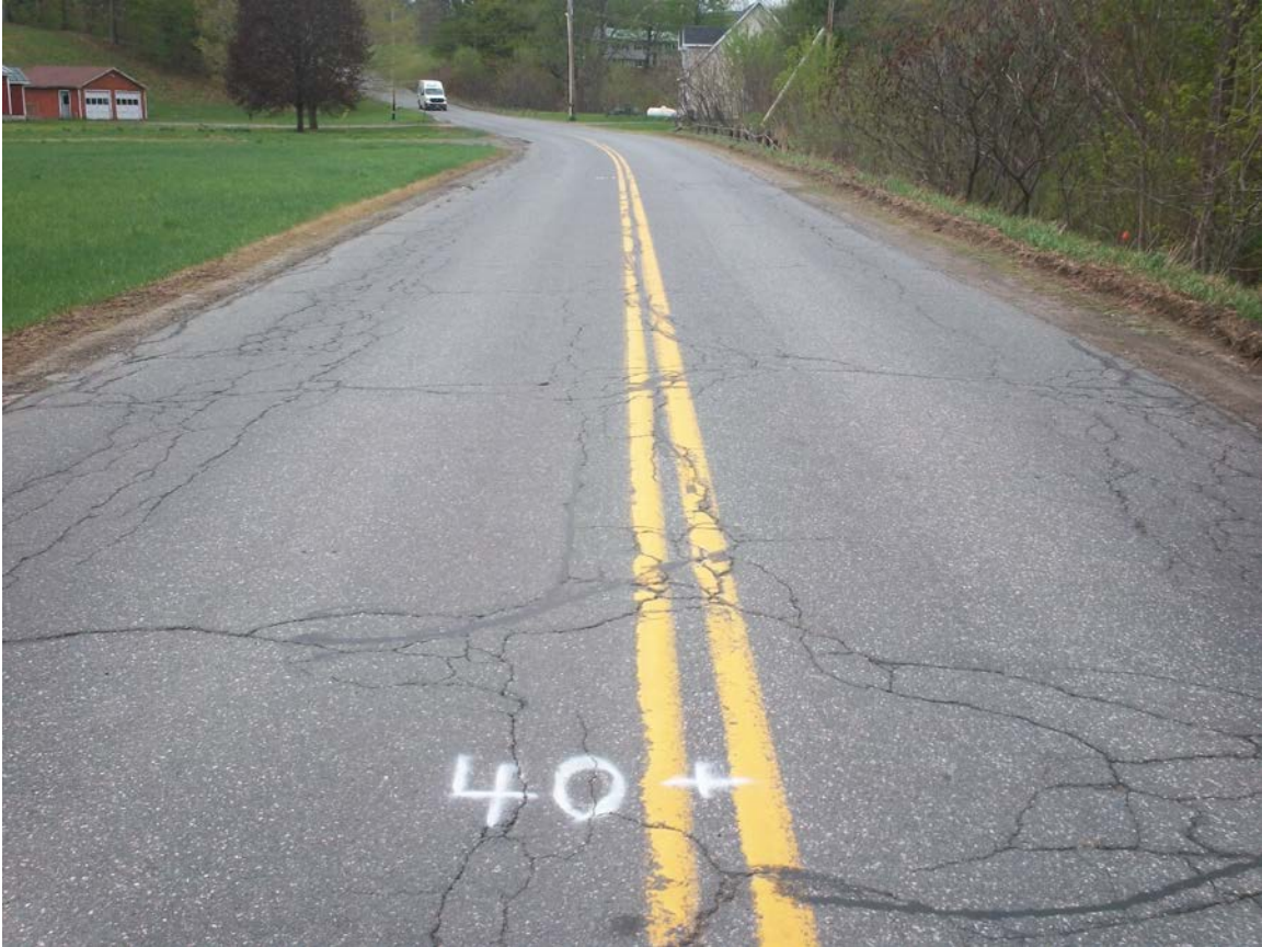
River Road: Photo taken 2015 at station 40+00 (before shim, overlay, chip seal).
