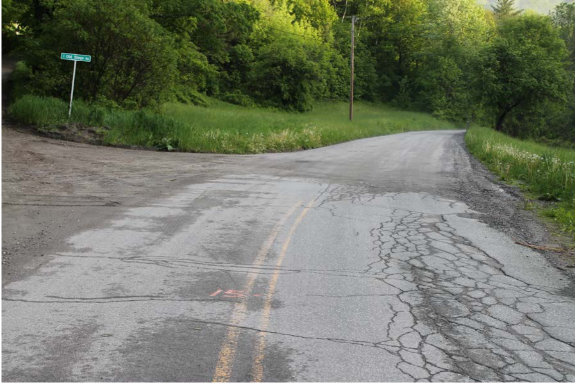
Broad Brook Road: Photo taken 5/31/2017 at station 15+00.
