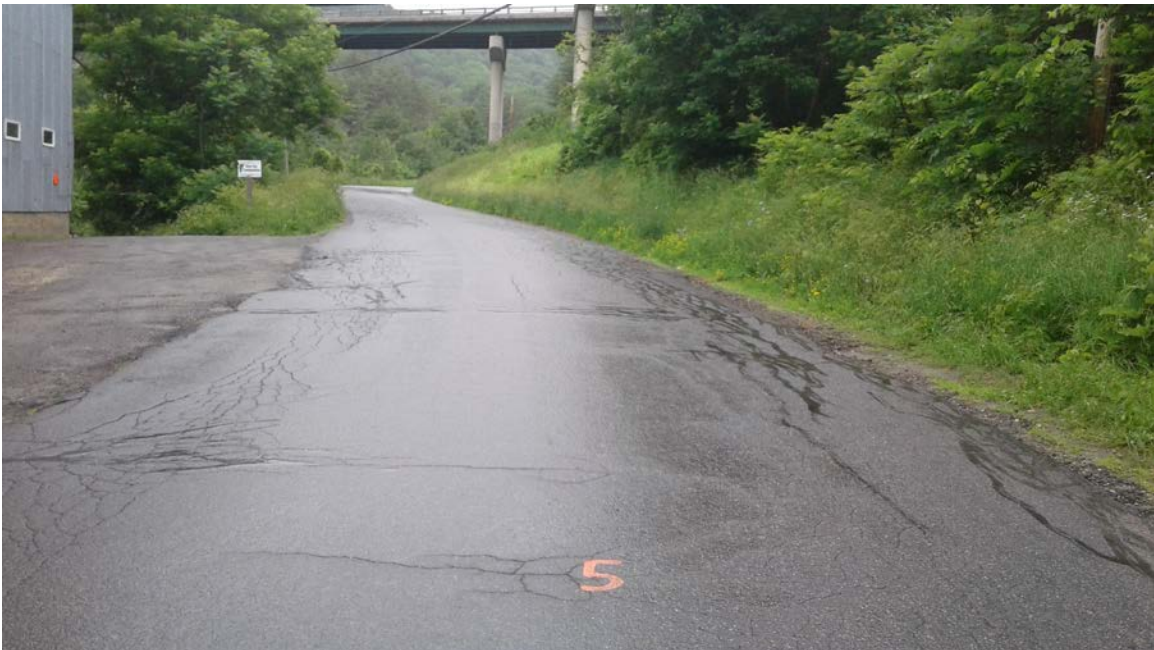
Fay Brook Road: Photo taken 6/29/2017 at station 5+00.
