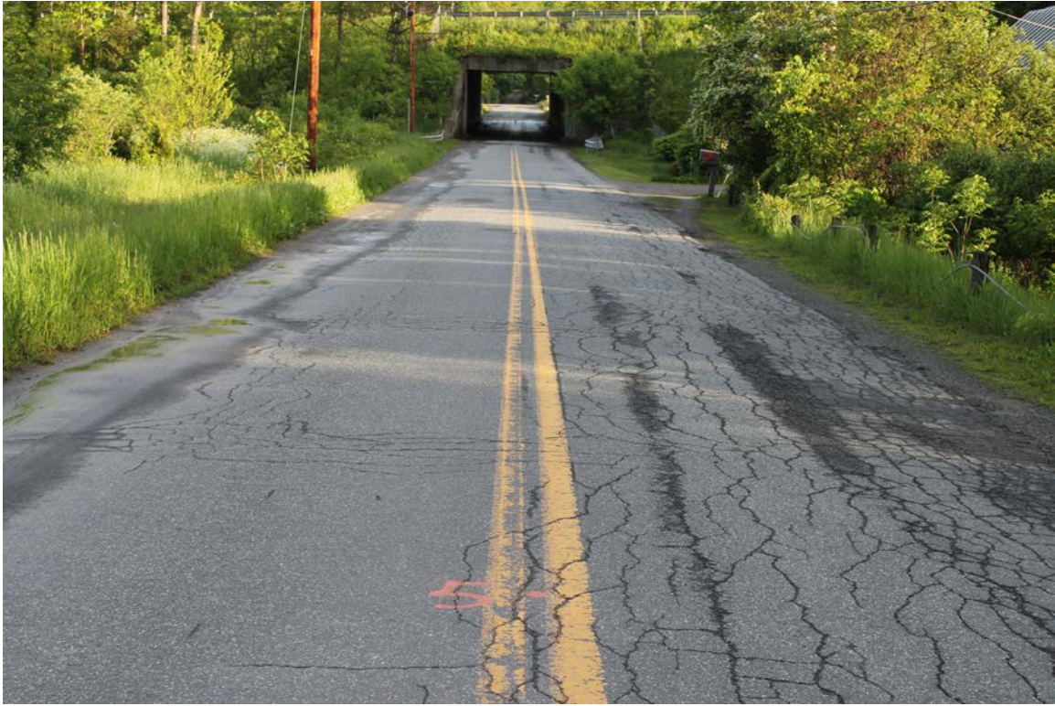
Broad Brook Road: Photo taken 5/31/2017 at station 5+00.
