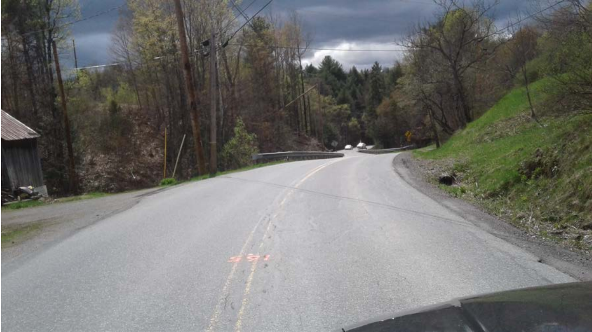
Rte #132: Photo taken 5/3/2017 at station 165+00.
