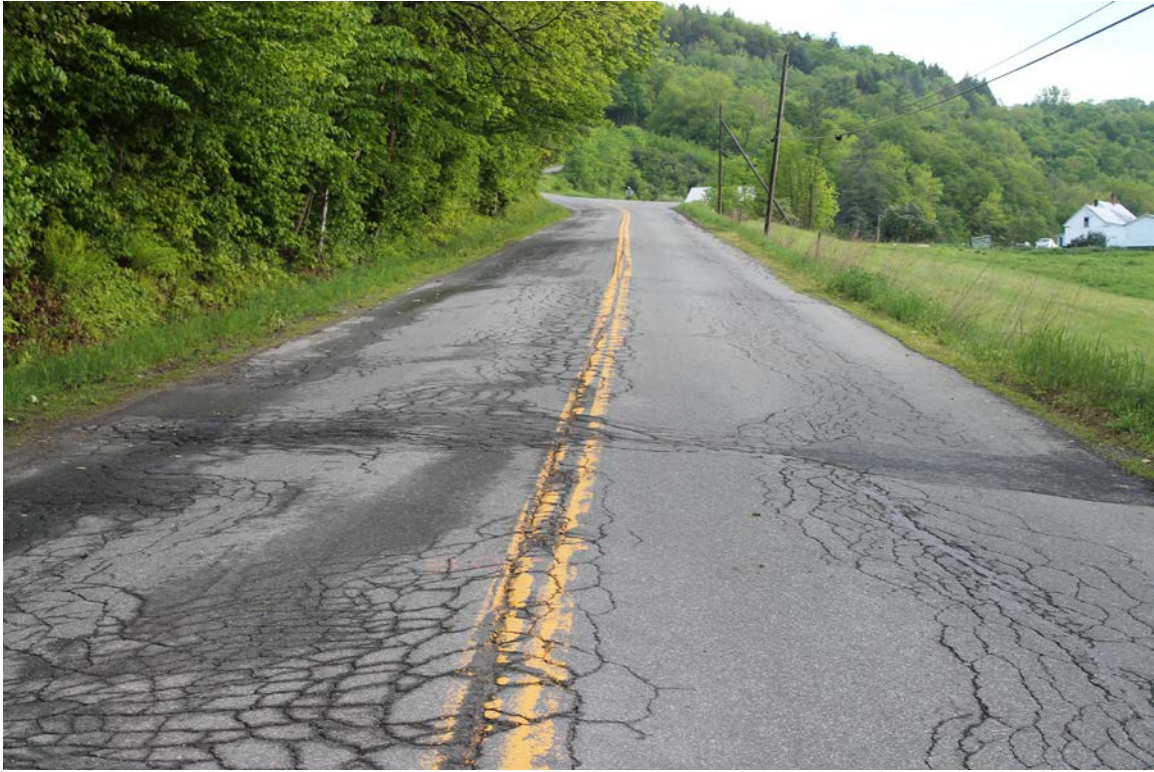
Howe Hill Road: Photo taken 5/31/2017 at station 30+00.
