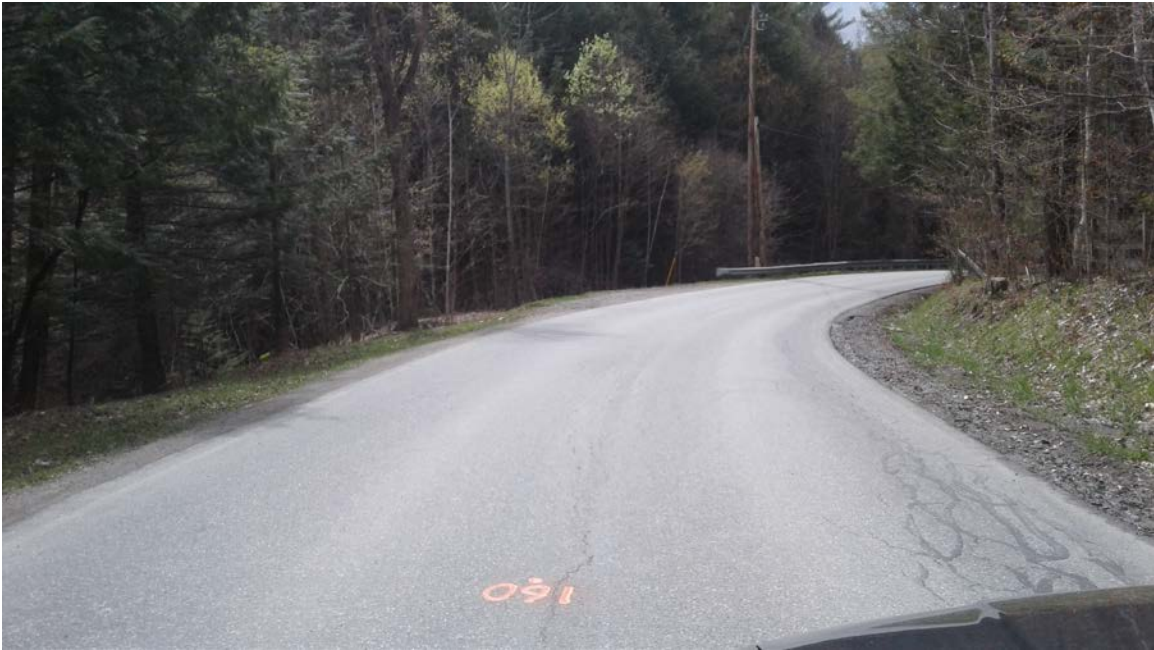
Rte #132: Photo taken 5/3/2017 at station 160+00.
