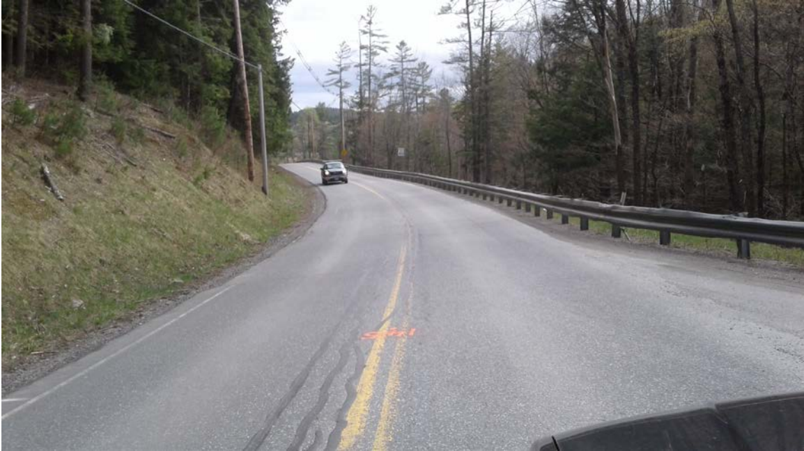
Rte #132: Photo taken 5/3/2017 at station 145+00.
