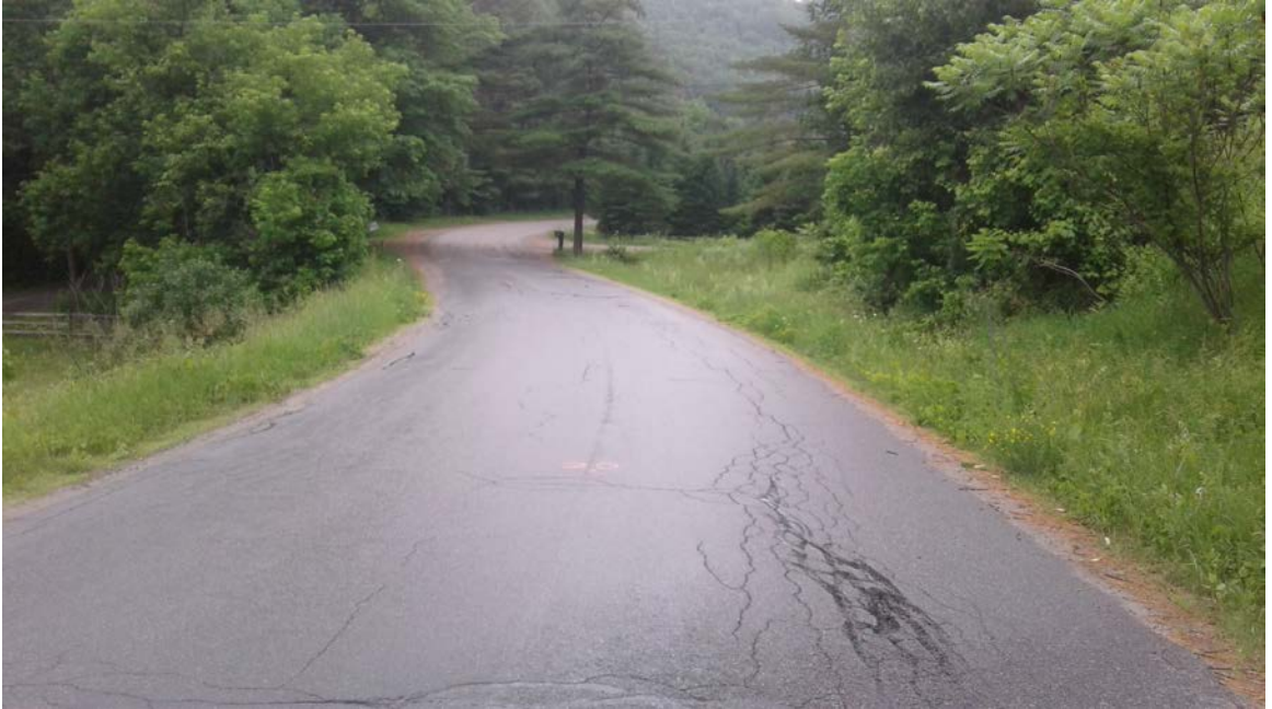
Fay Brook Road: Photo taken 6/29/2017 at station 20+00.
