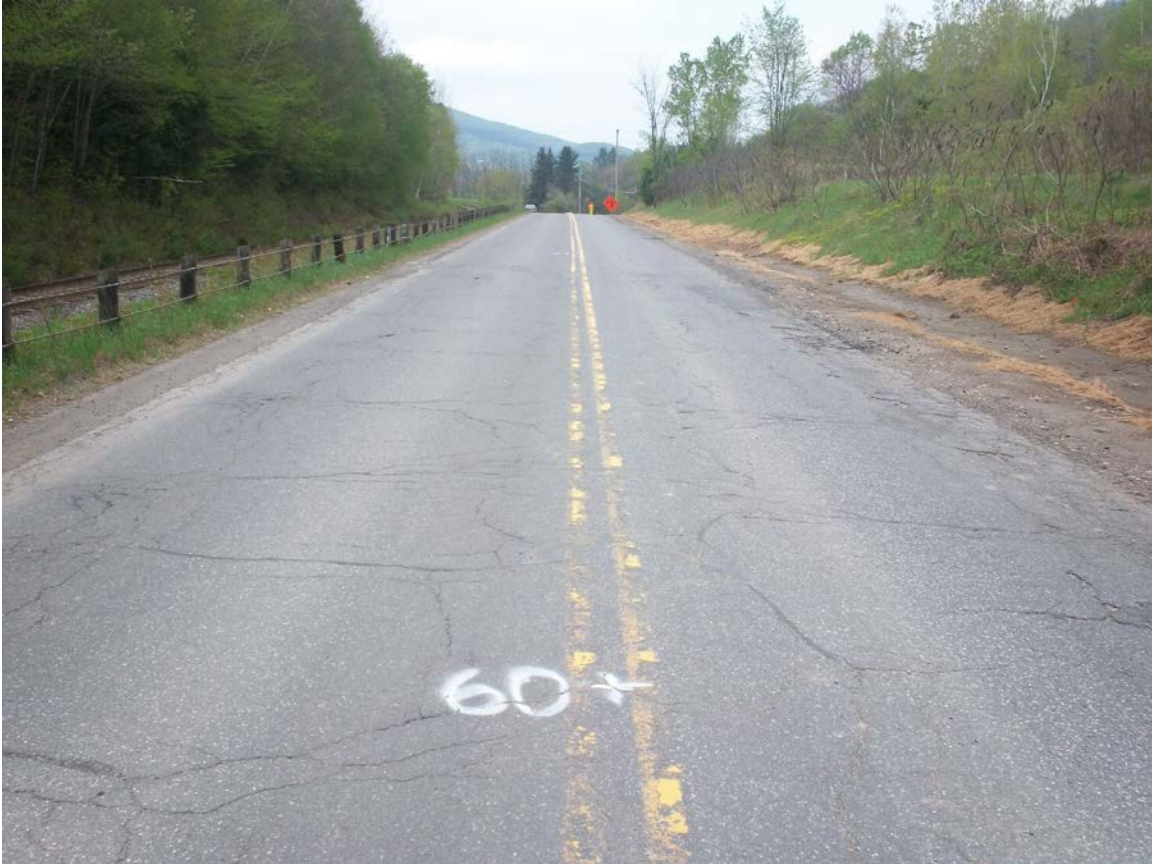
River Road: Photo taken 2015 at station 60+00 (before shim, overlay, chip seal).
