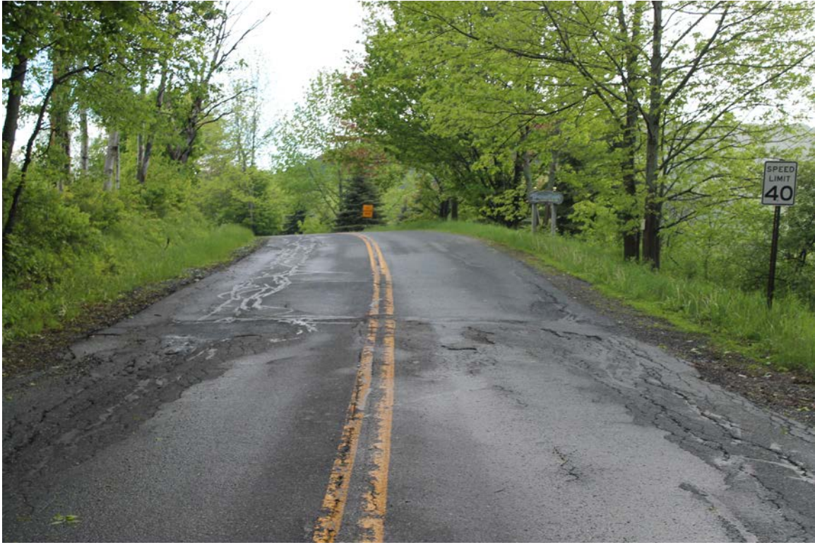
Howe Hill Road: Photo taken 5/31/2017 at station 143+60.
