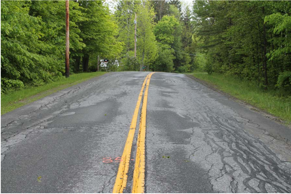
Howe Hill Road: Photo taken 5/31/2017 at station 85+00.
