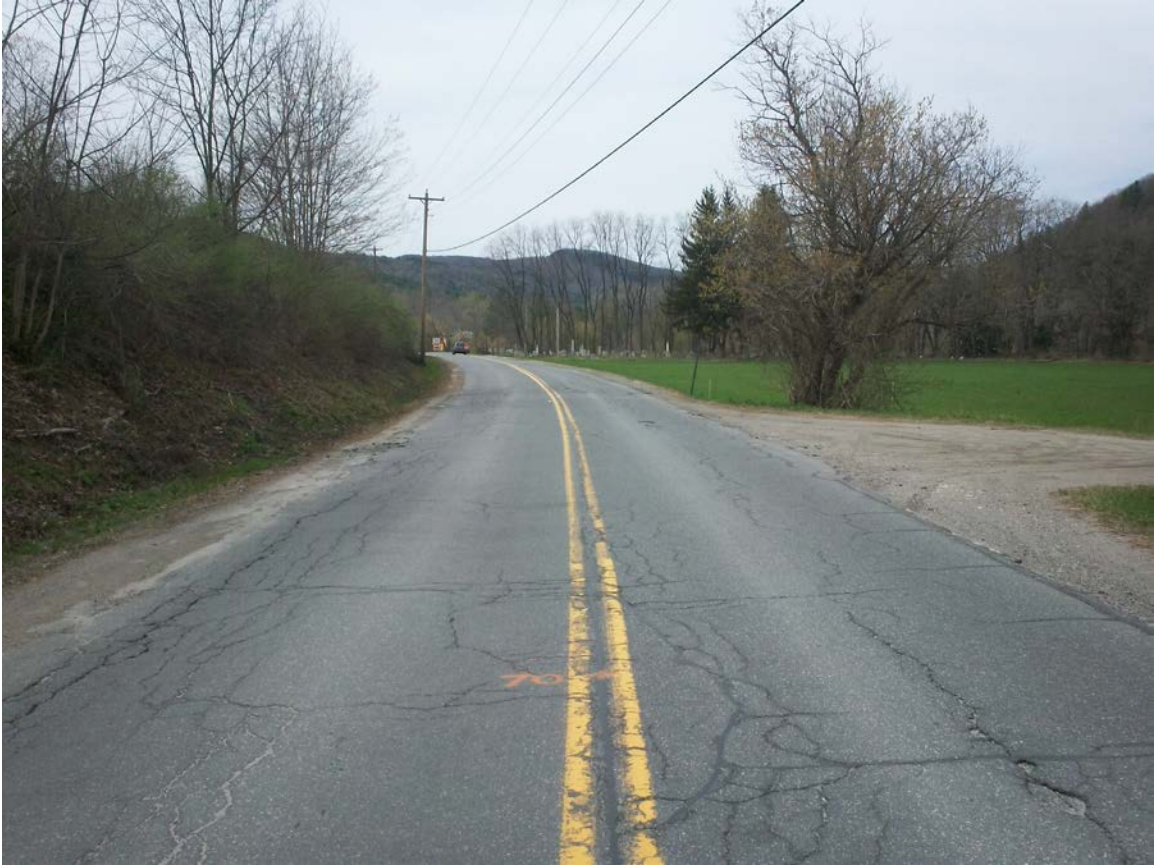
River Road: Photo taken 2015 at station 70+00 (before shim, overlay, chip seal).
