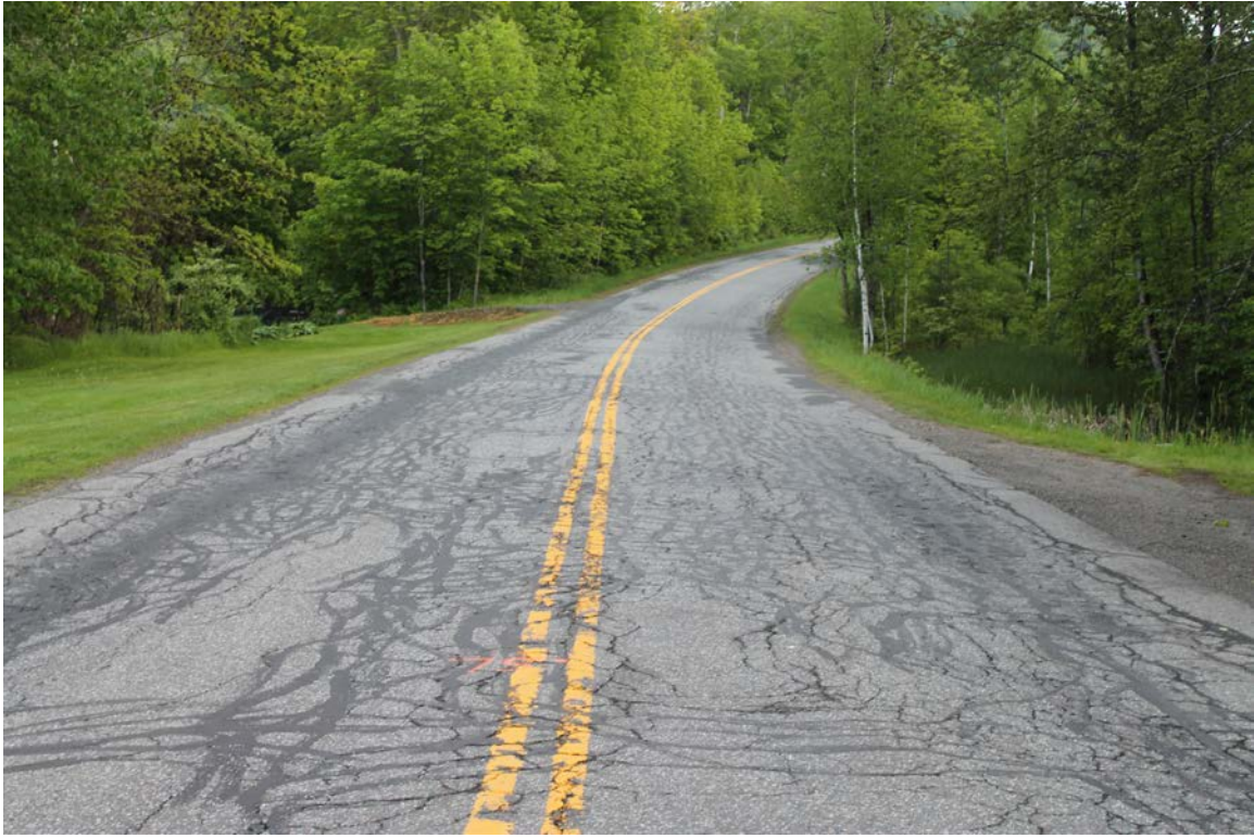
Howe Hill Road: Photo taken 5/31/2017 at station 75+00.
