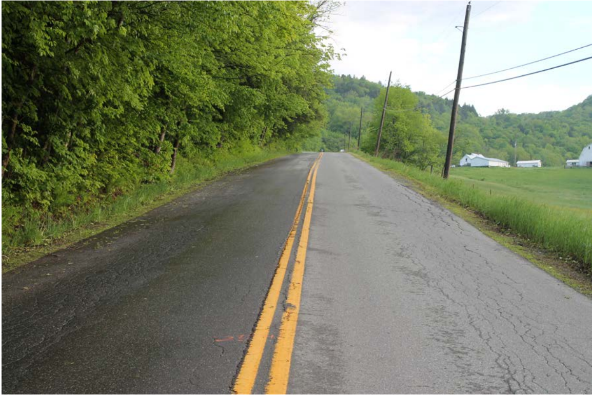
Howe Hill Road: Photo taken 5/31/2017 at station 25+00.
