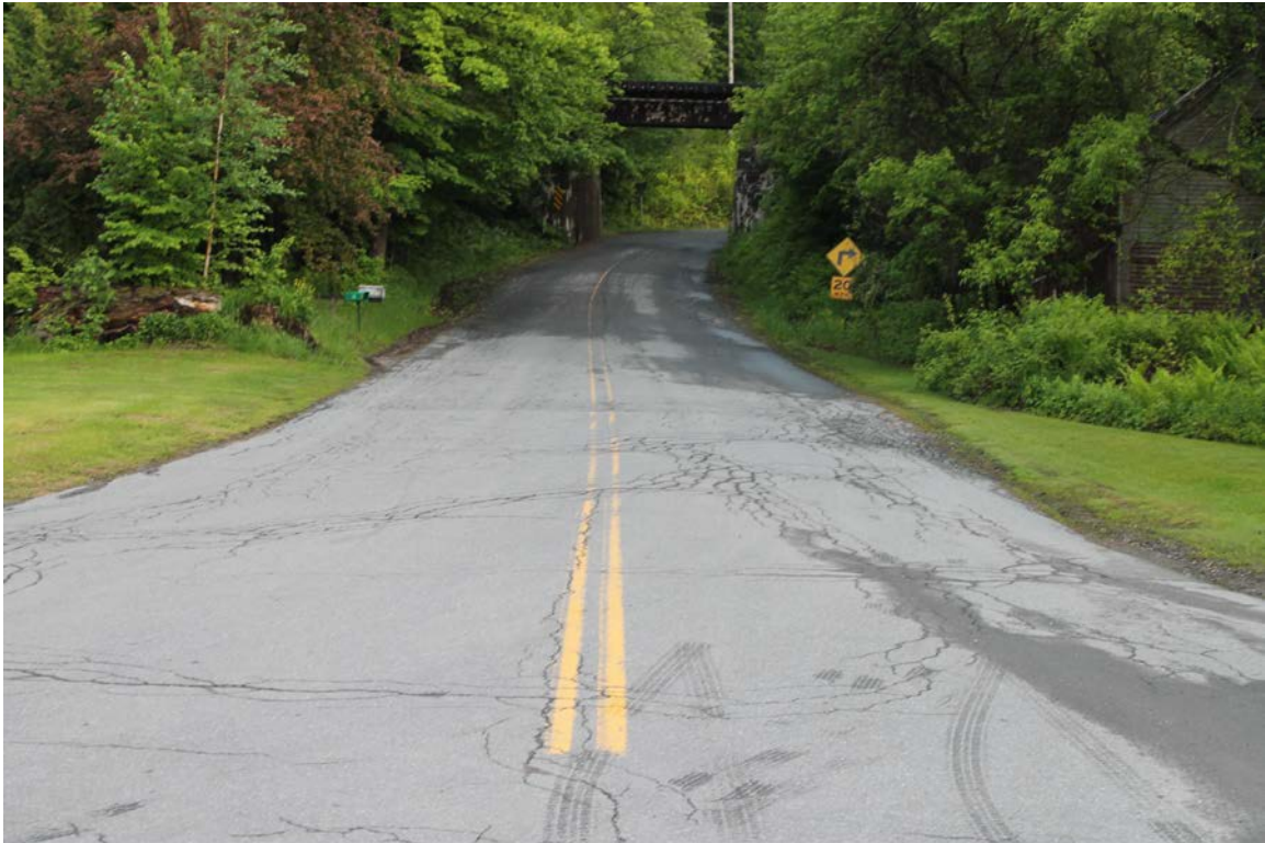
Howe Hill Road: Photo taken 5/31/2017 at station 0+00.
