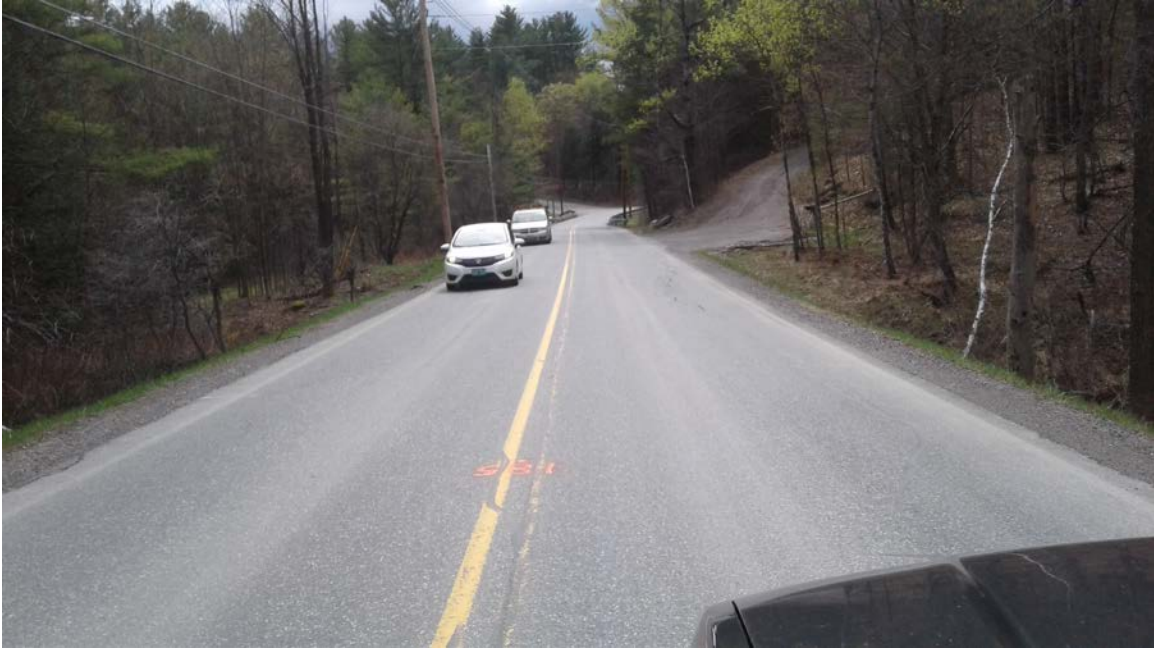
Rte #132: Photo taken 5/3/2017 at station 185+00.
