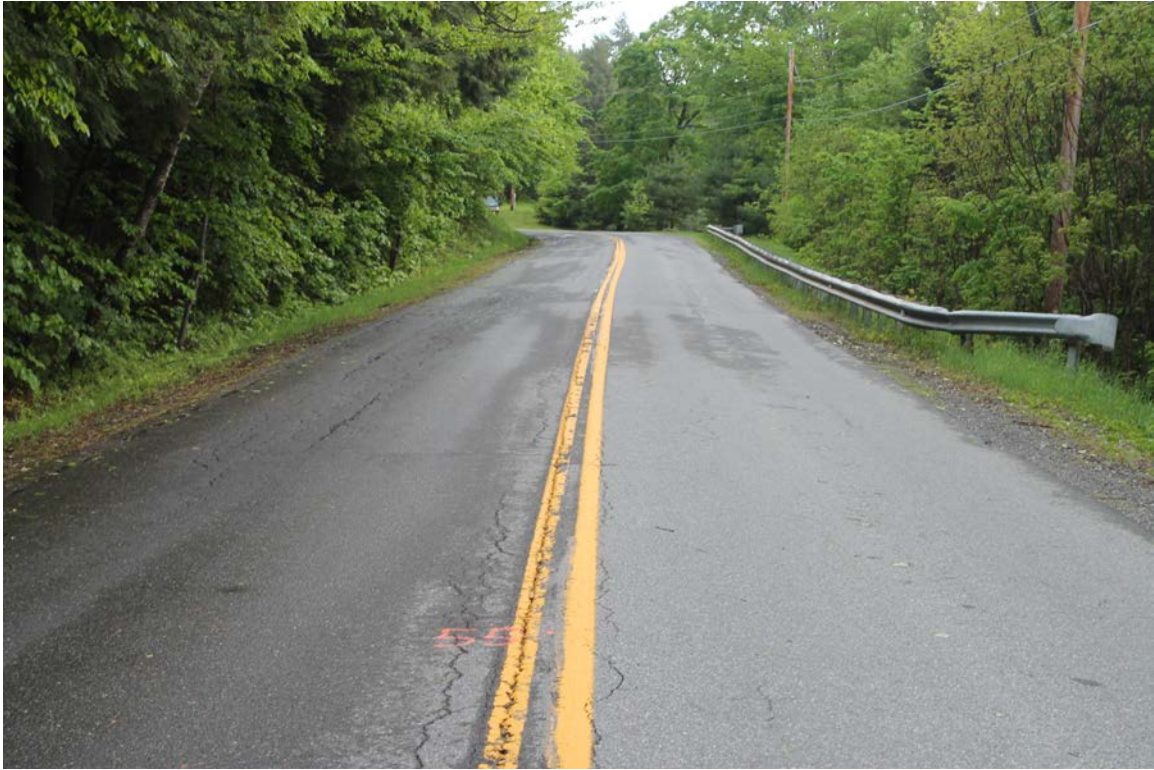
Howe Hill Road: Photo taken 5/31/2017 at station 55+00.
