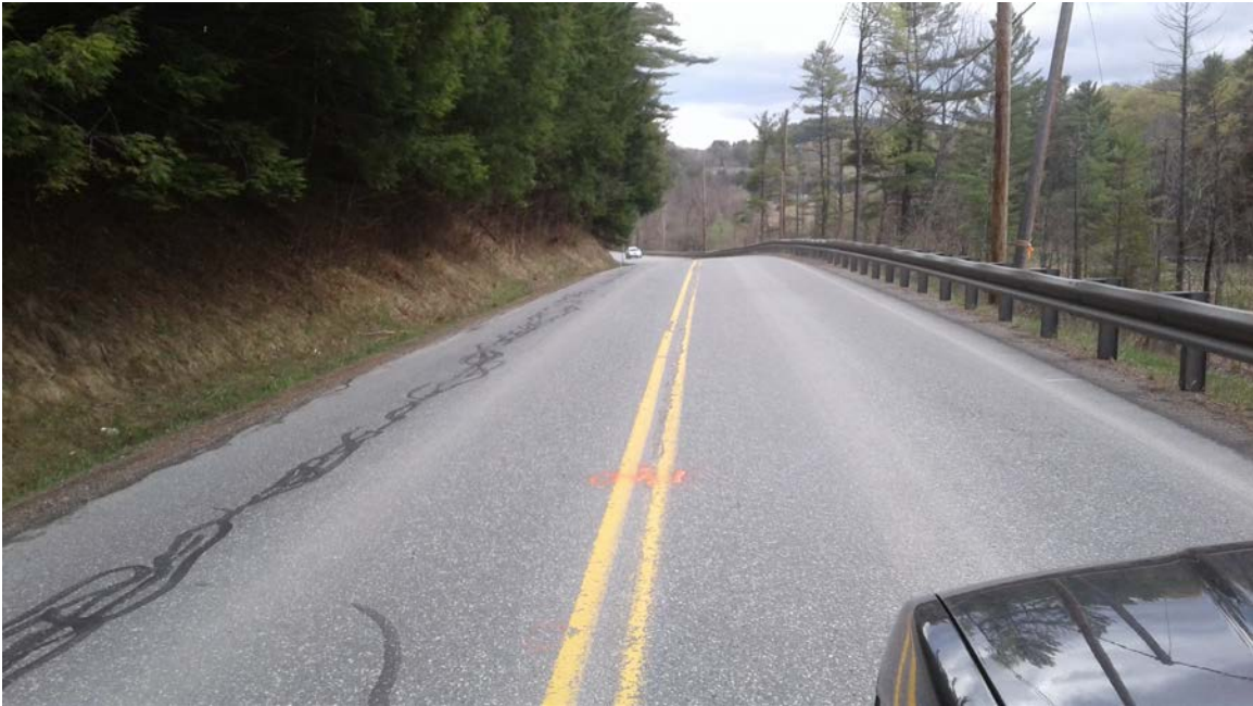
Rte #132: Photo taken 5/3/2017 at station 140+00.
