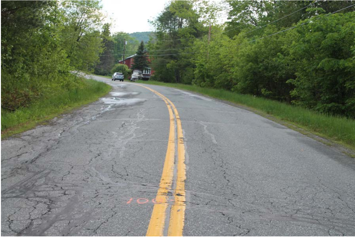
Howe Hill Road: Photo taken 5/31/2017 at station 100+00.
