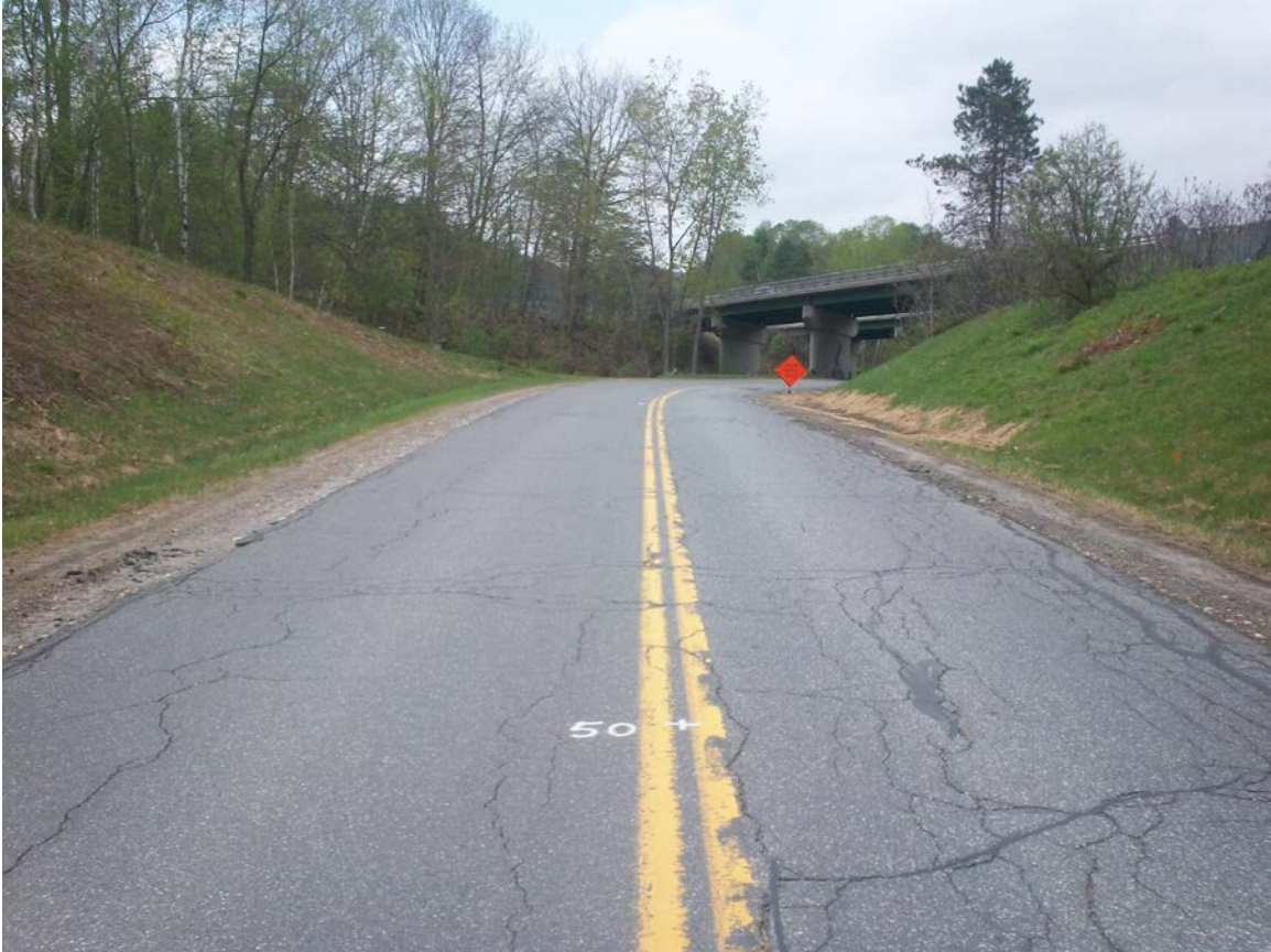
River Road: Photo taken 2015 at station 50+00 (before shim, overlay, chip seal).
