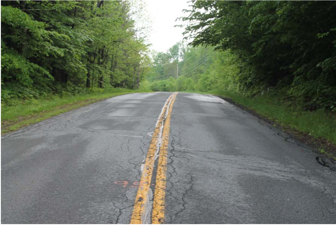
Howe Hill Road: Photo taken 5/31/2017 at station 95+00.
