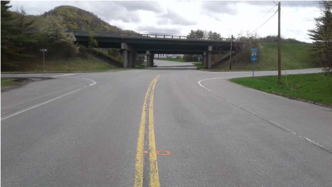
Rte #132: Photo taken 5/3/2017 at station 0+00.
