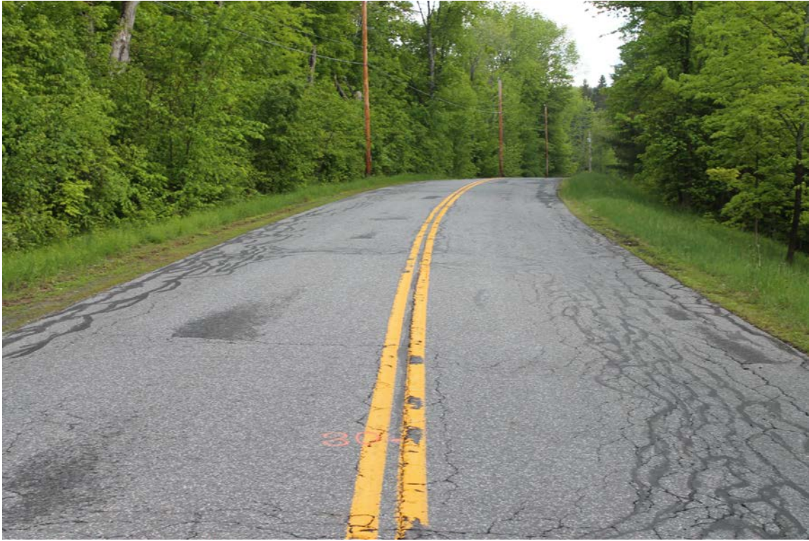
Howe Hill Road: Photo taken 5/31/2017 at station 80+00.
