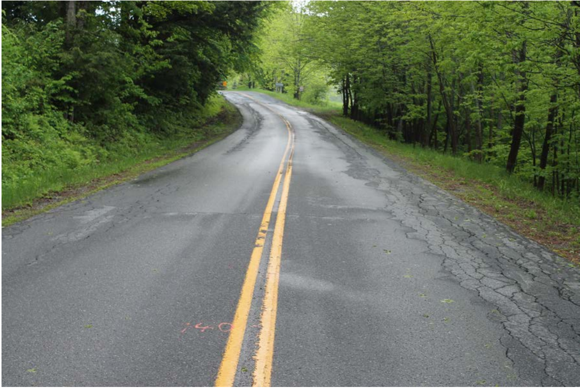
Howe Hill Road: Photo taken 5/31/2017 at station 140+00.
