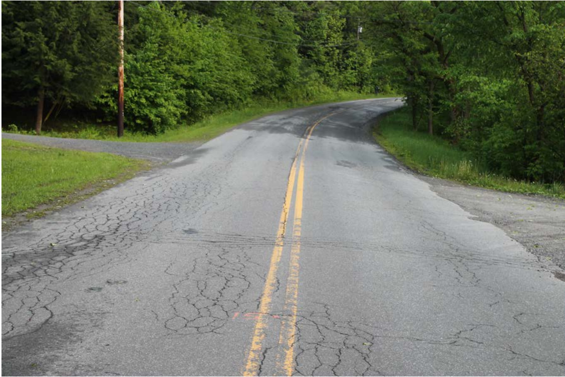
Howe Hill Road: Photo taken 5/31/2017 at station 15+00.
