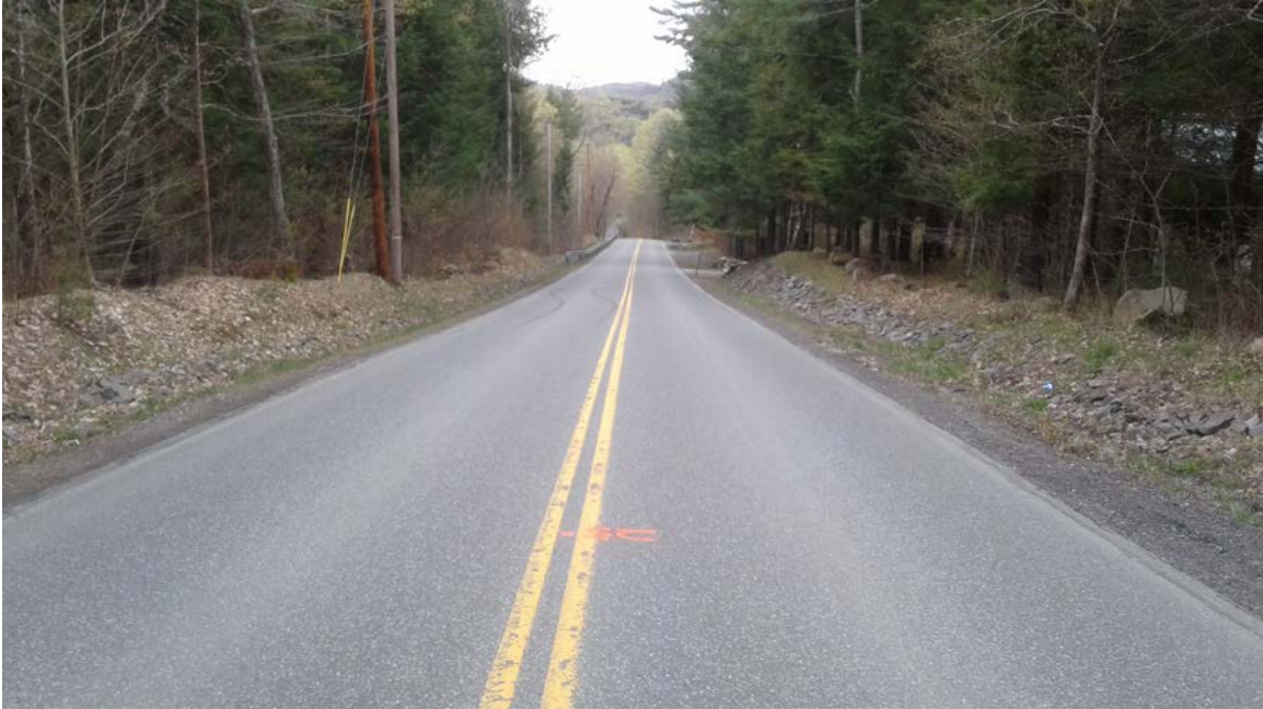
Rte #132: Photo taken 5/3/2017 at station 25+00.
