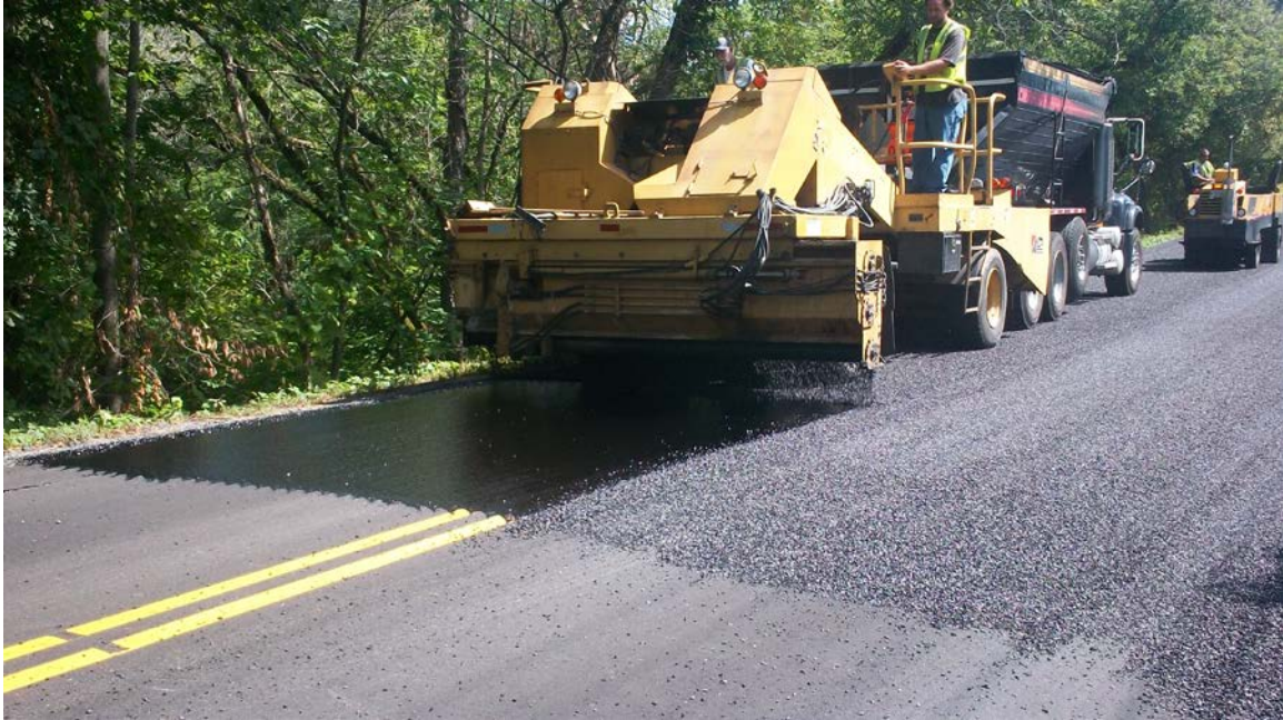
River Road: Photo taken 2015 during chip sealing with 10% rubber.
