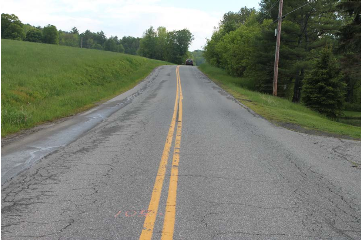
Howe Hill Road: Photo taken 5/31/2017 at station 105+00.
