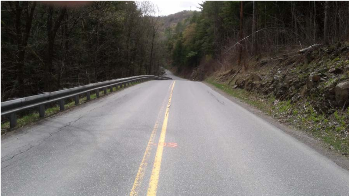
Rte #132: Photo taken 5/3/2017 at station 50+00.
