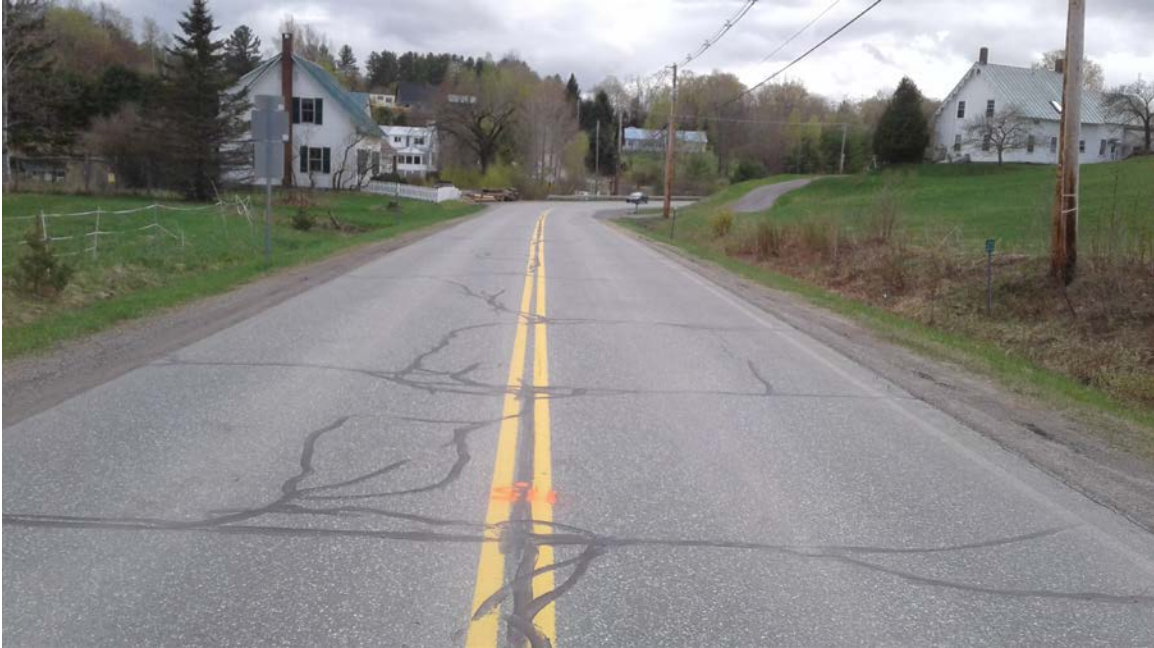
Rte #132: Photo taken 5/3/2017 at station 115+00.
