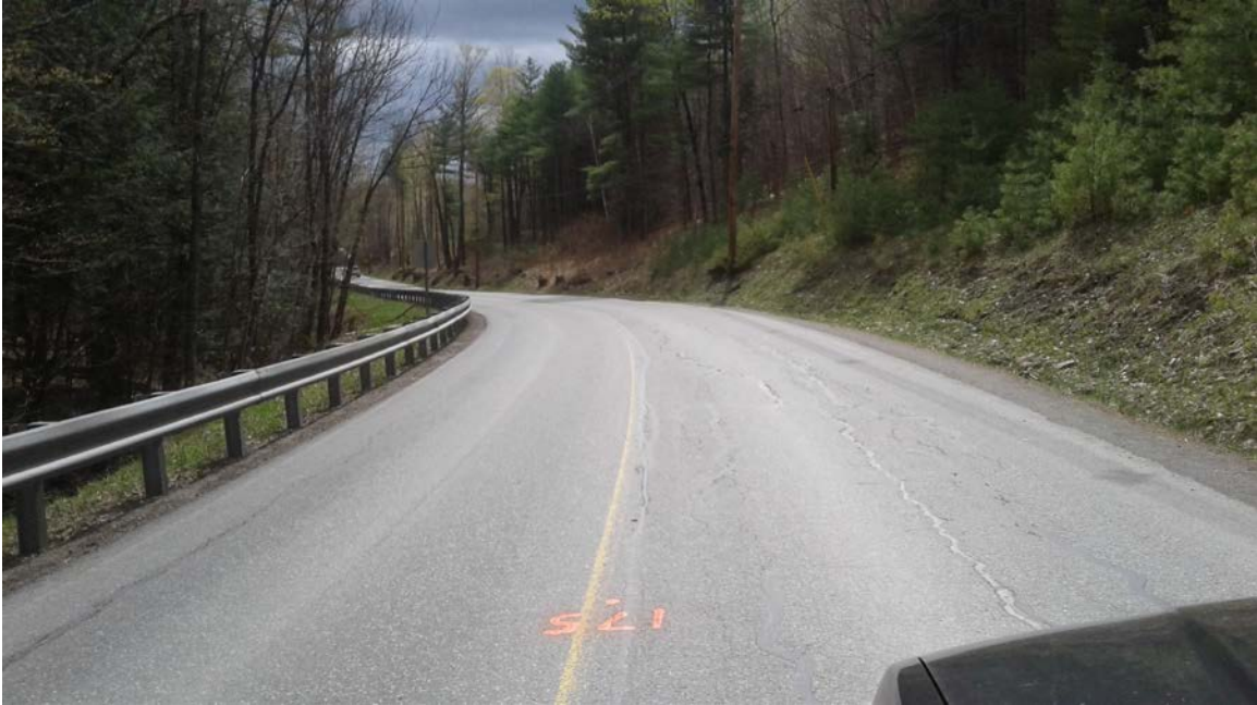
Rte #132: Photo taken 5/3/2017 at station 175+00.
