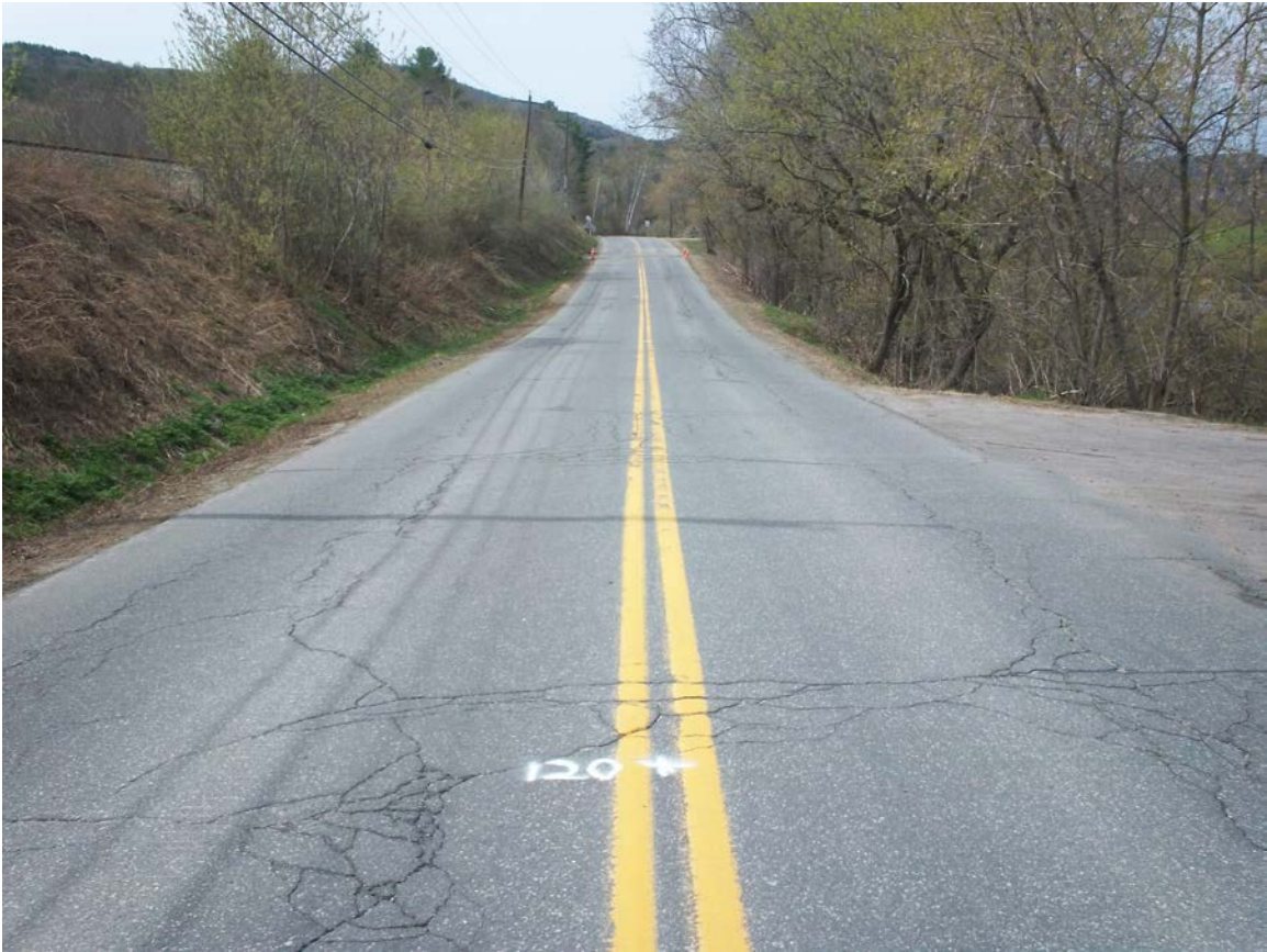
River Road: Photo taken 2015 at station 120+00 (before shim, overlay, chip seal).
