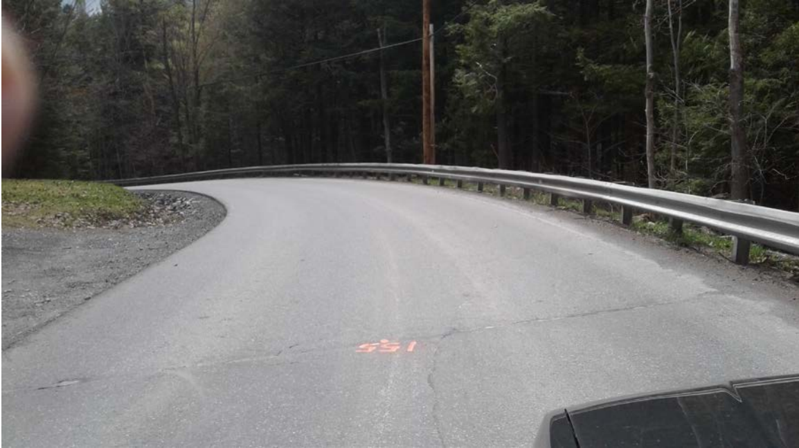
Rte #132: Photo taken 5/3/2017 at station 155+00.
