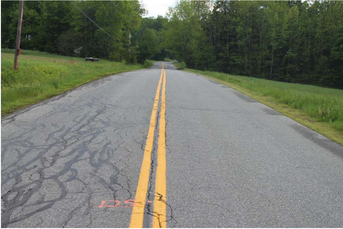
Howe Hill Road: Photo taken 5/31/2017 at station 125+00.
