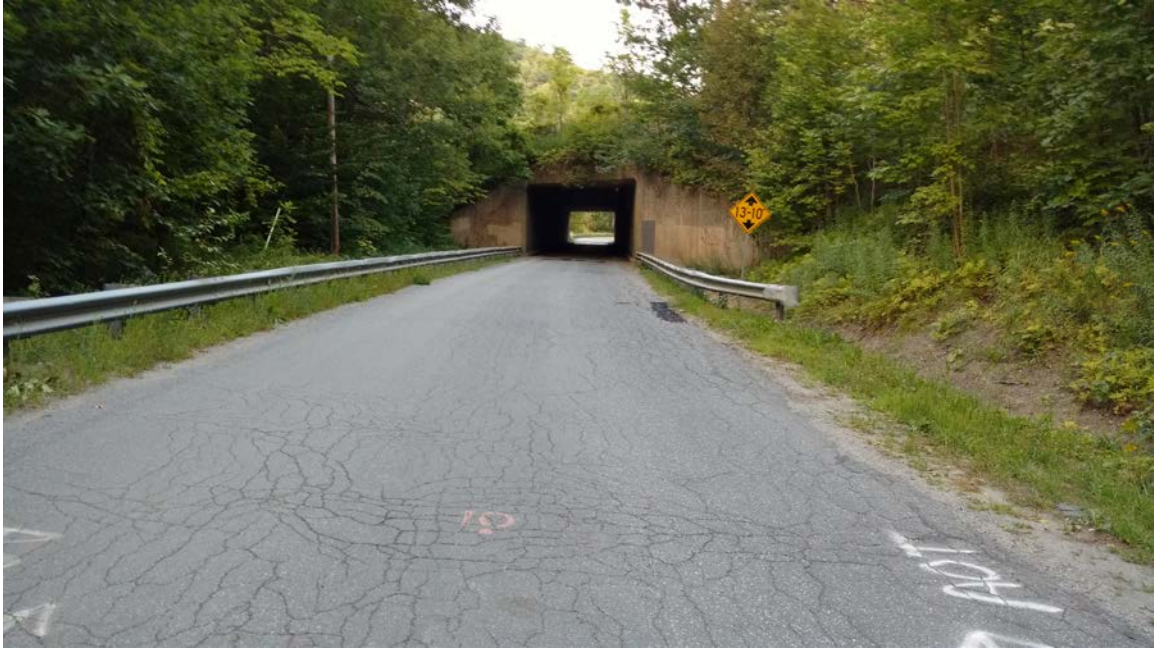
Quimby Mountain Road: Photo taken 8/31/2017 at station 10+00.
