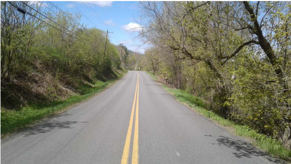
River Road: Photo taken 5/11/2017 at station 120+00.
