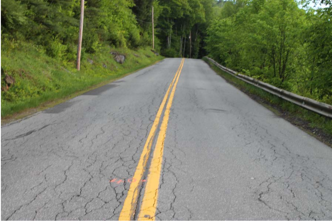
Howe Hill Road: Photo taken 5/31/2017 at station 40+00.
