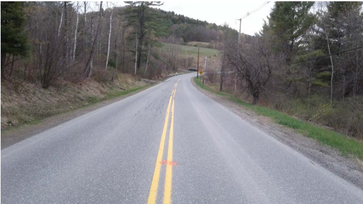
Rte #132: Photo taken 5/3/2017 at station 90+00.
