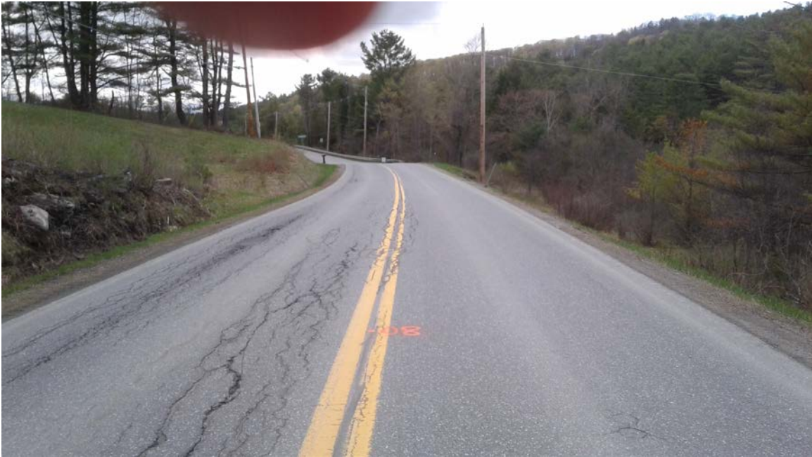
Rte #132: Photo taken 5/3/2017 at station 80+00.
