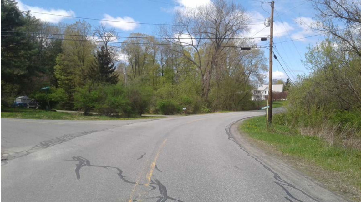
River Road: Photo taken 5/11/2017 at station 30+00.
