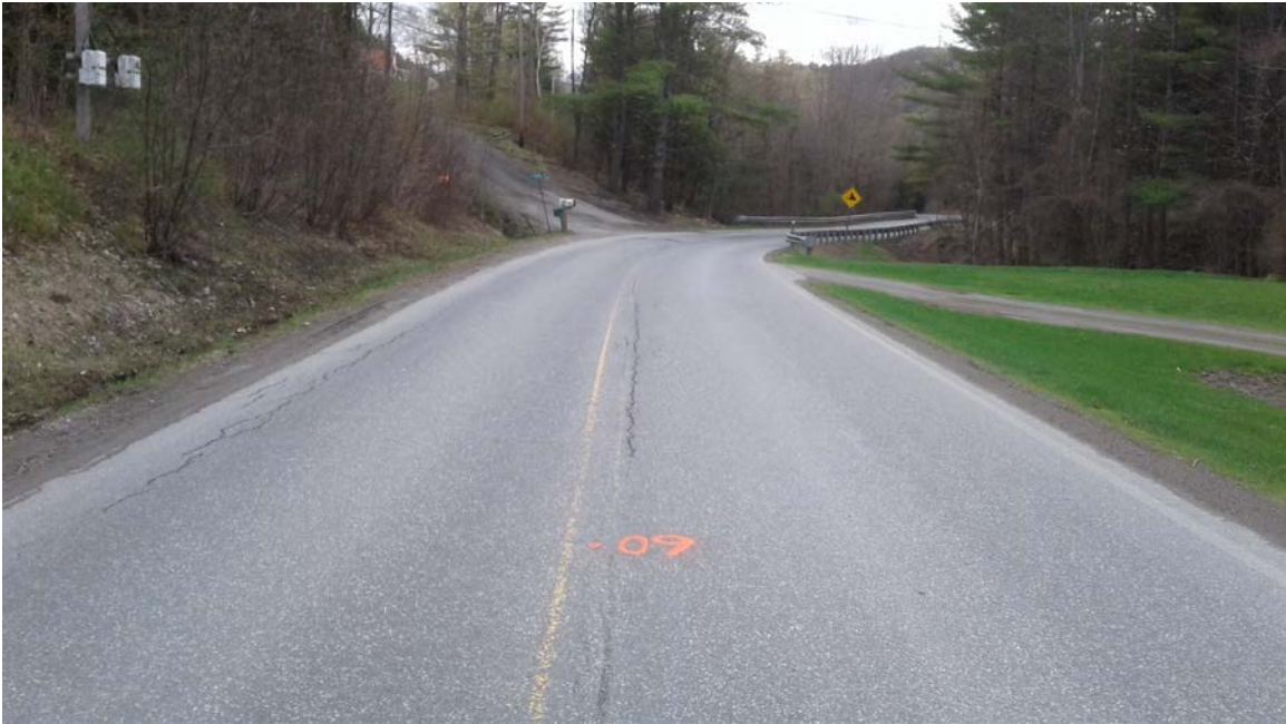
Rte #132: Photo taken 5/3/2017 at station 60+00.
