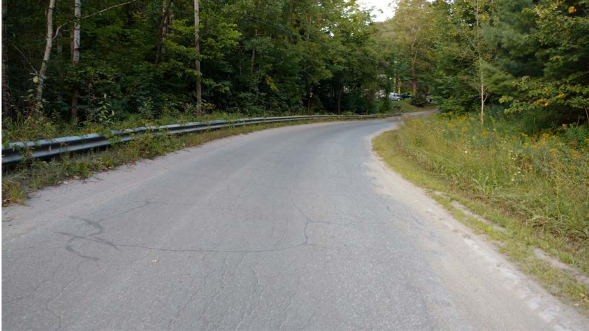
Quimby Mountain Road: Photo taken 8/31/2017 at station 17+00.
