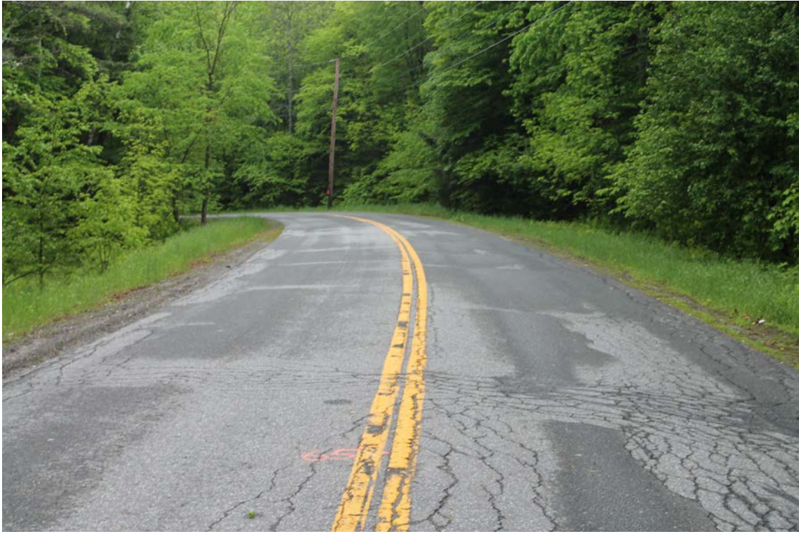
Howe Hill Road: Photo taken 5/31/2017 at station 65+00.
