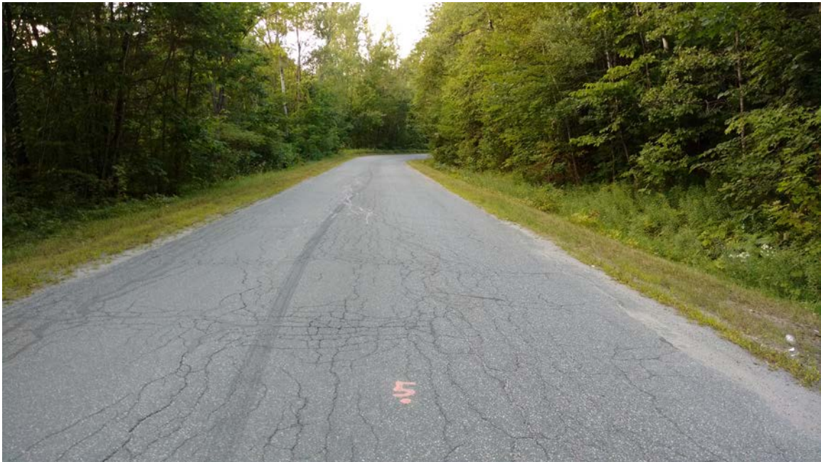
Quimby Mountain Road: Photo taken 8/31/2017 at station 5+00.
