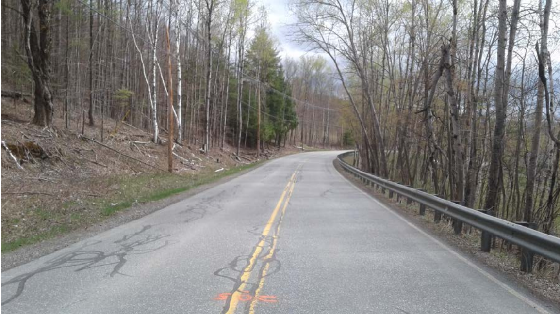
Rte #132: Photo taken 5/3/2017 at station 205+00.
