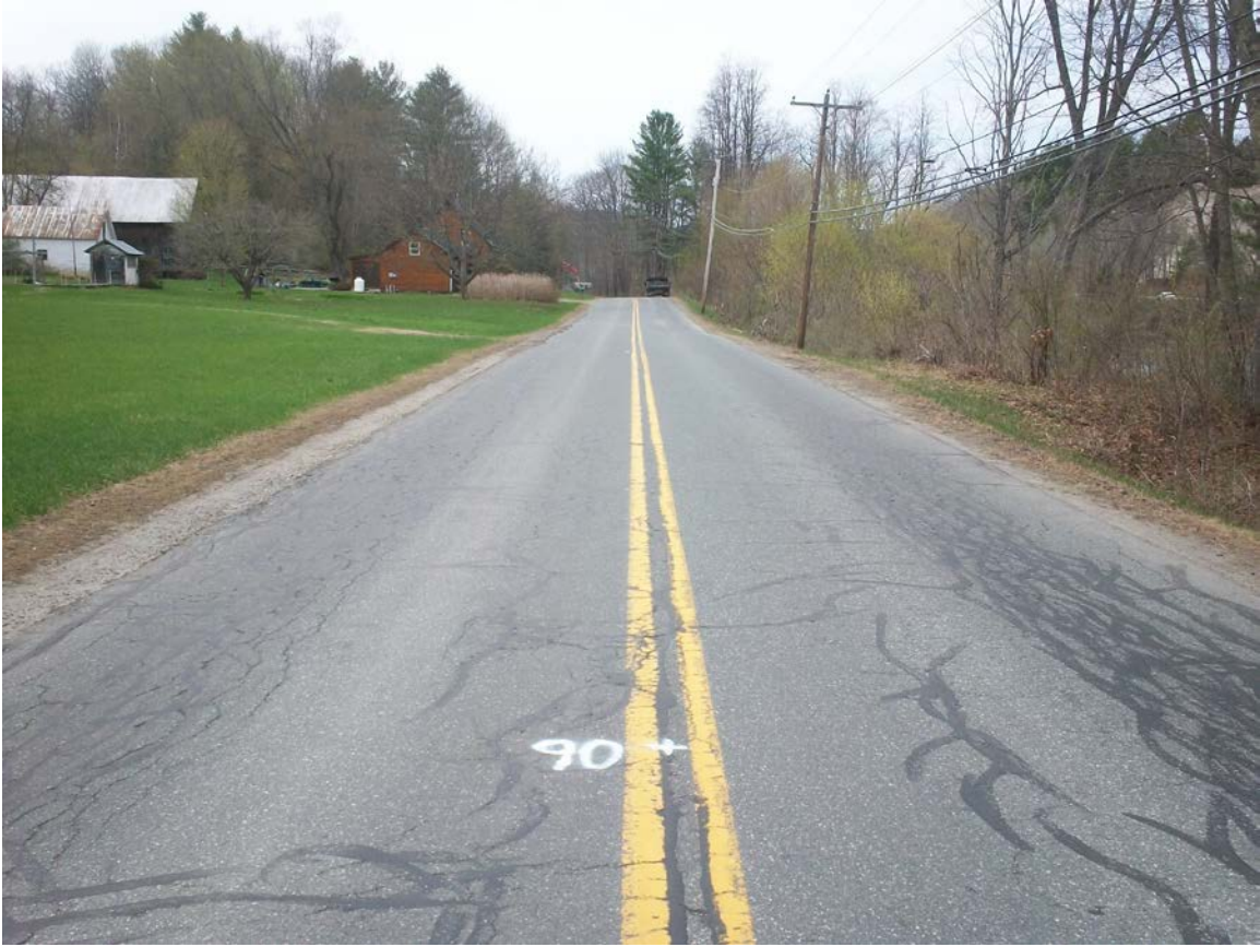
River Road: Photo taken 2015 at station 90+00 (before shim, overlay, chip seal).
