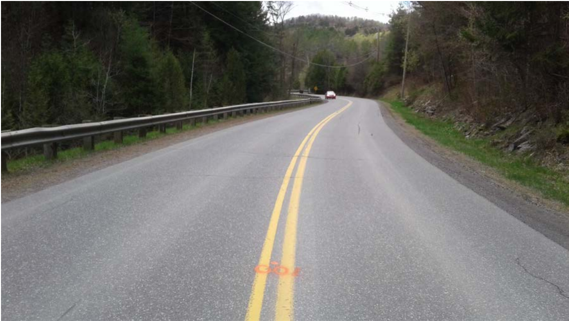
Rte #132: Photo taken 5/3/2017 at station 100+00.
