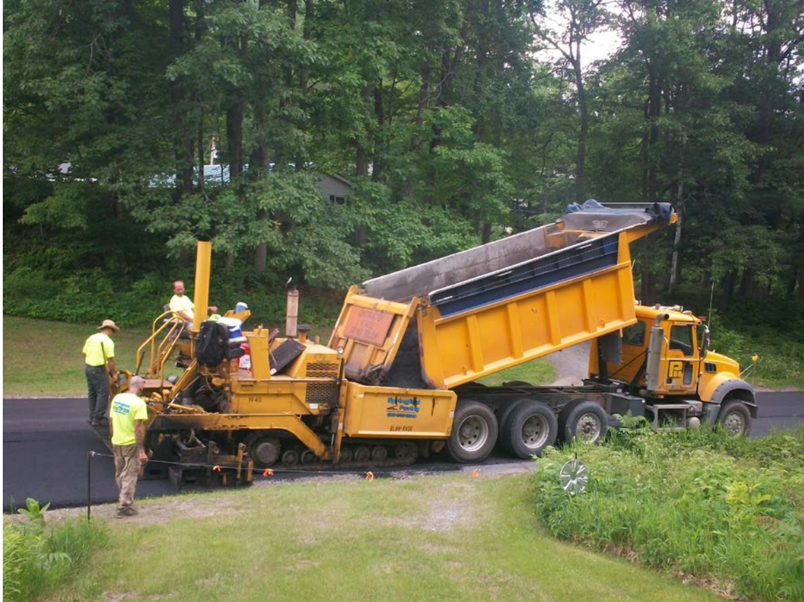
River Road: Photo taken 2015 during an asphalt overlay (Station 33+00 to 126+10).
