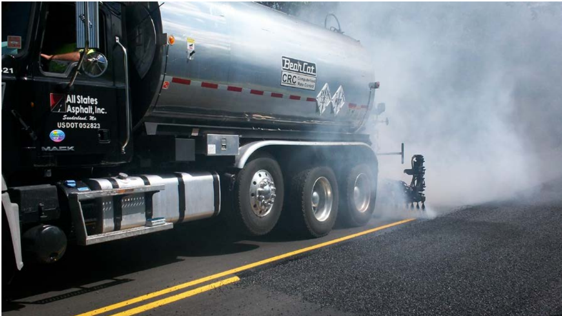
River Road: Photo taken 2015 during chip sealing with 10% rubber.
