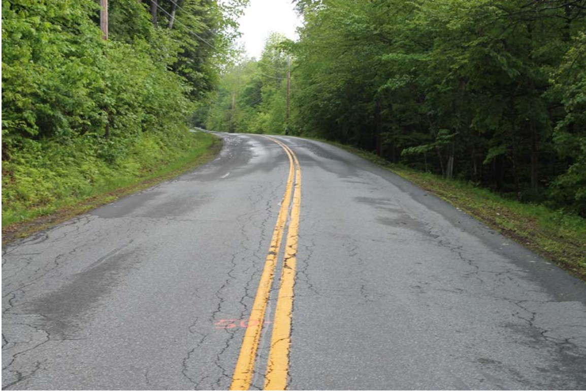
Howe Hill Road: Photo taken 5/31/2017 at station 50+00.
