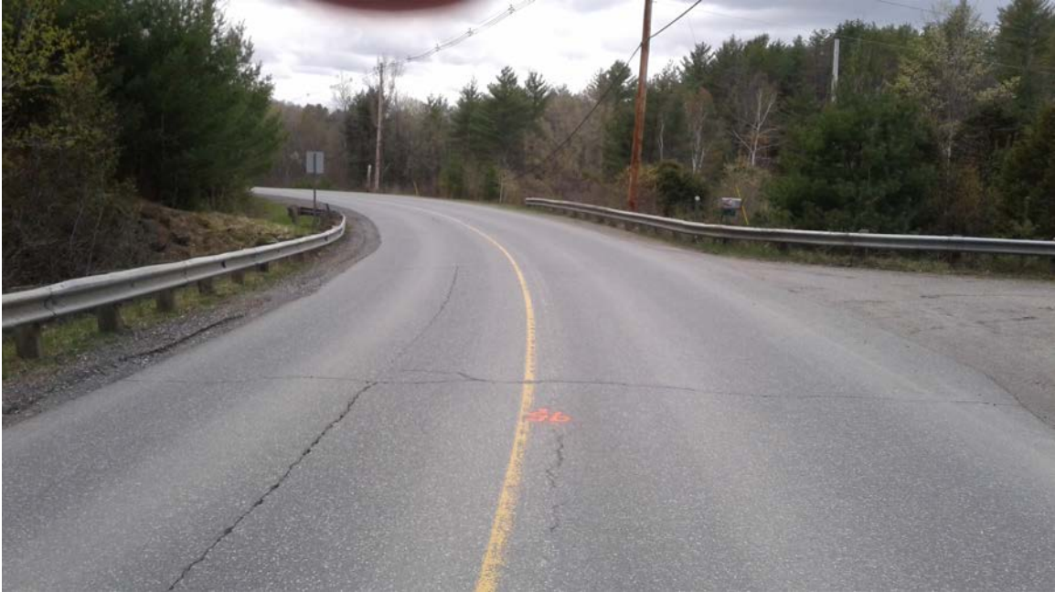
Rte #132: Photo taken 5/3/2017 at station 95+00.
