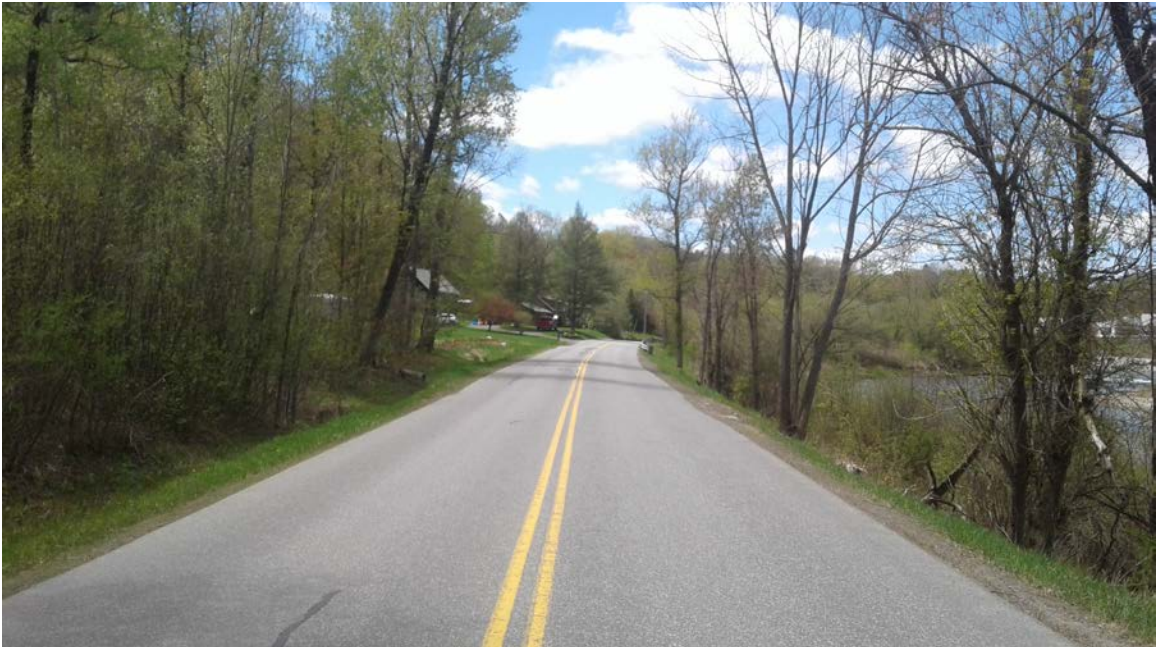
River Road: Photo taken 5/11/2017 at station 20+00.
