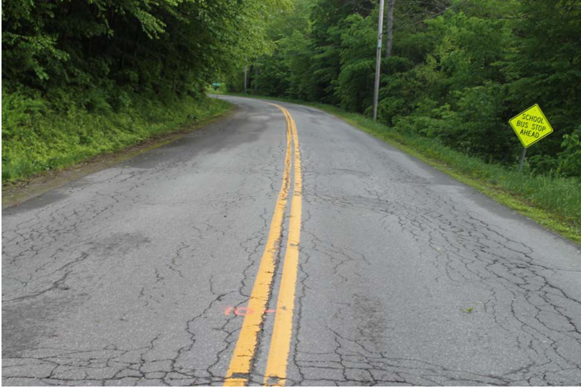
Howe Hill Road: Photo taken 5/31/2017 at station 10+00.
