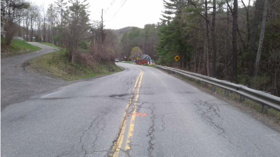
Rte #132: Photo taken 5/3/2017 at station 65+00.
