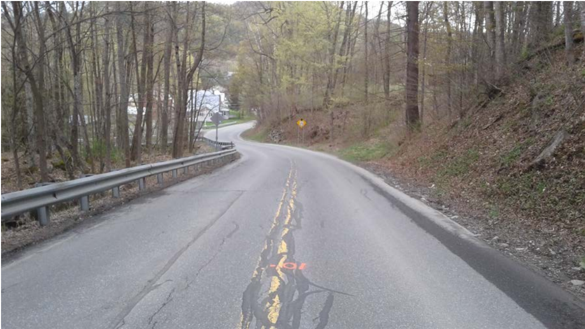
Rte #132: Photo taken 5/3/2017 at station 10+00.
