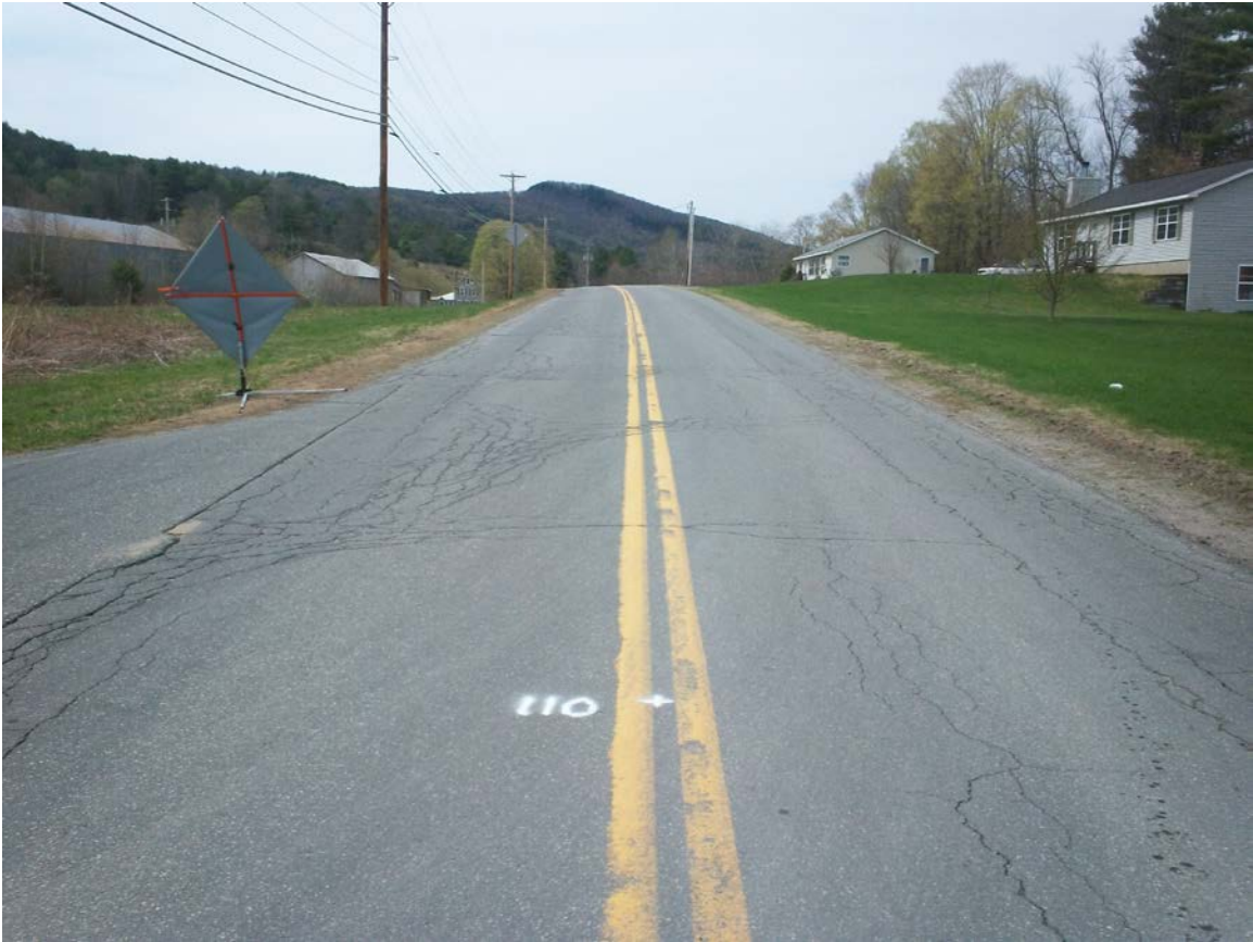
River Road: Photo taken 2015 at station 110+00 (before shim, overlay, chip seal).
