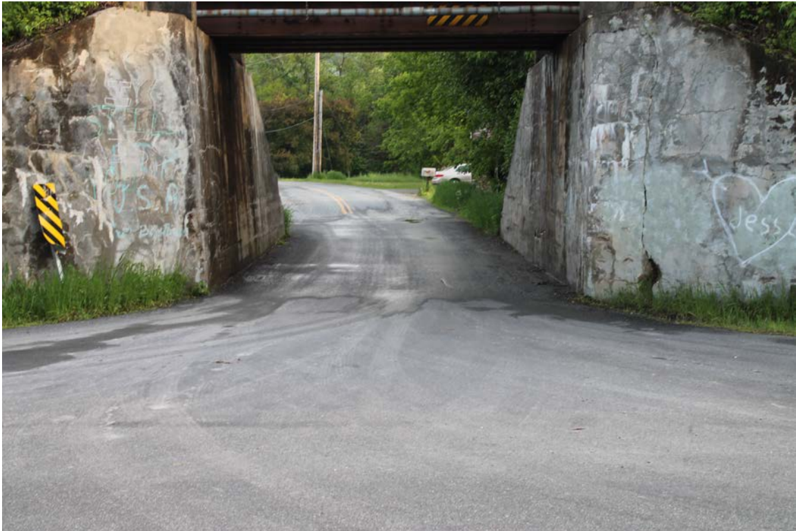
Broad Brook Road: Photo taken 5/31/2017 at station 0+00.
