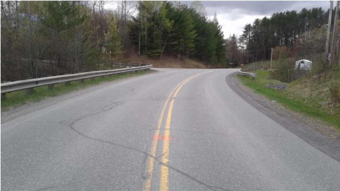
Rte #132: Photo taken 5/3/2017 at station 110+00.
