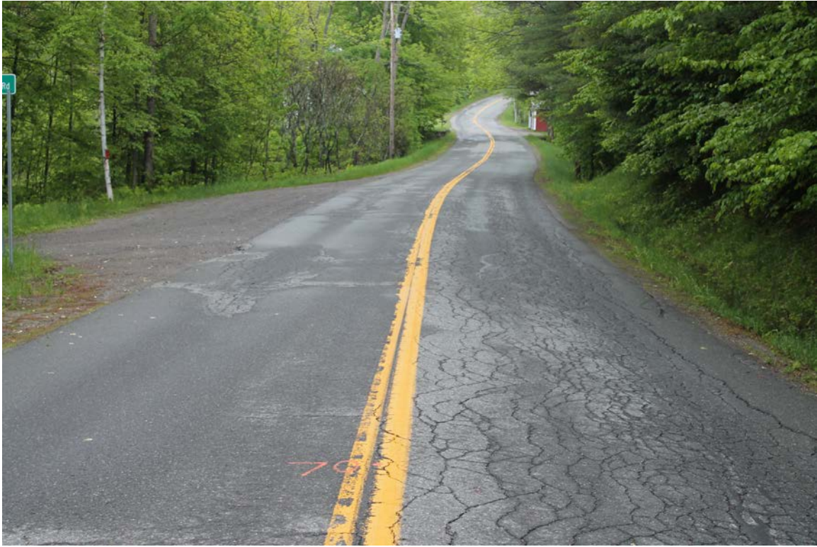
Howe Hill Road: Photo taken 5/31/2017 at station 70+00.
