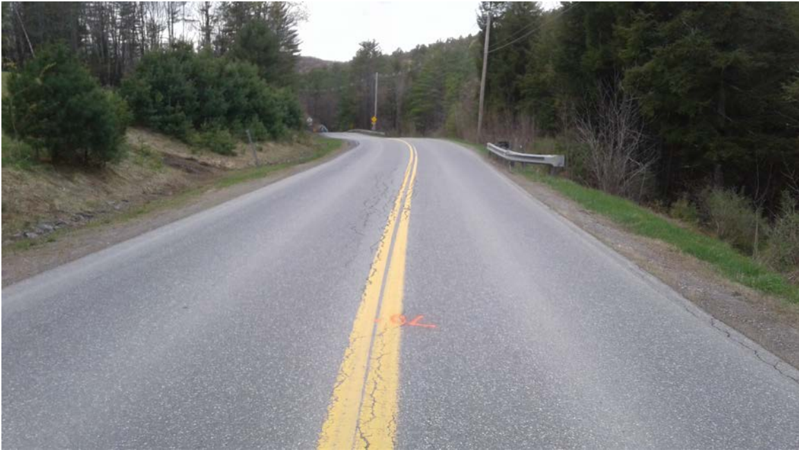
Rte #132: Photo taken 5/3/2017 at station 70+00.
