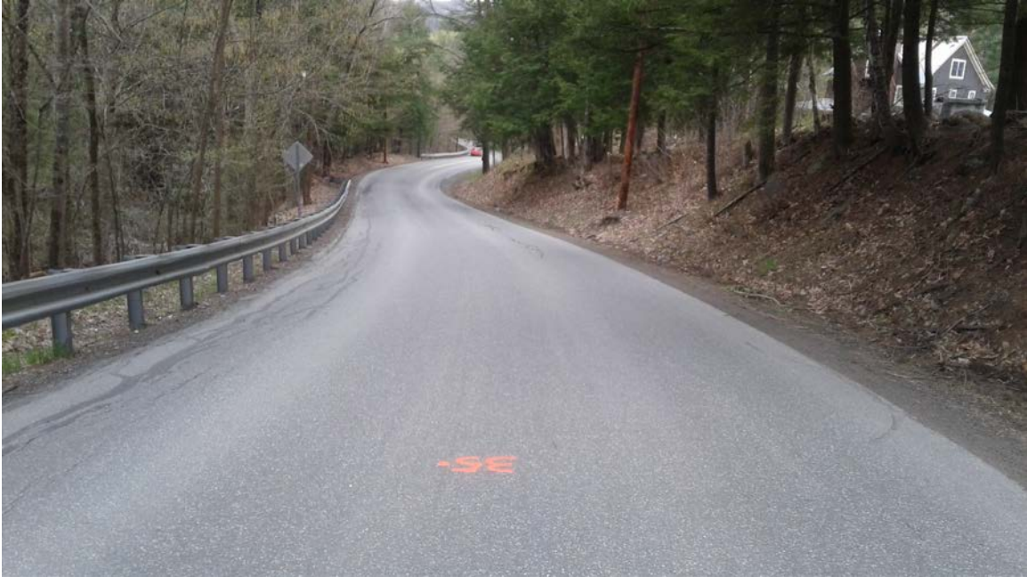
Rte #132: Photo taken 5/3/2017 at station 35+00.
