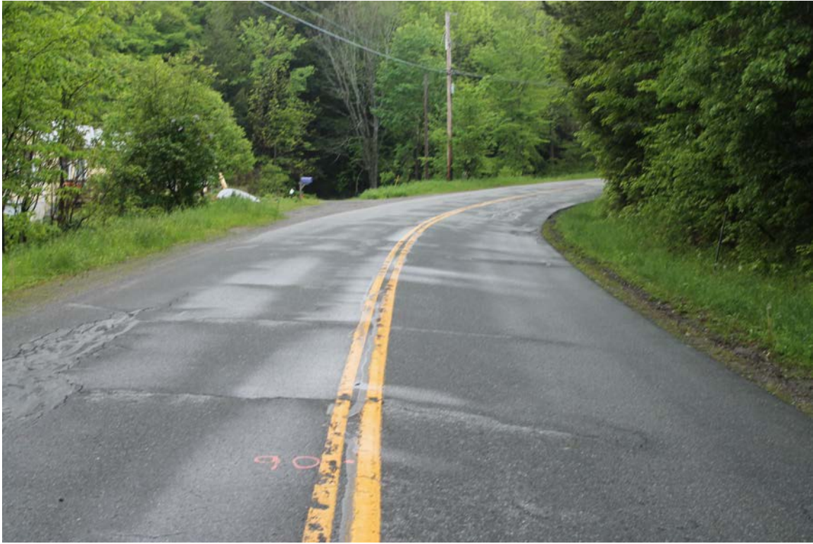
Howe Hill Road: Photo taken 5/31/2017 at station 90+00.
