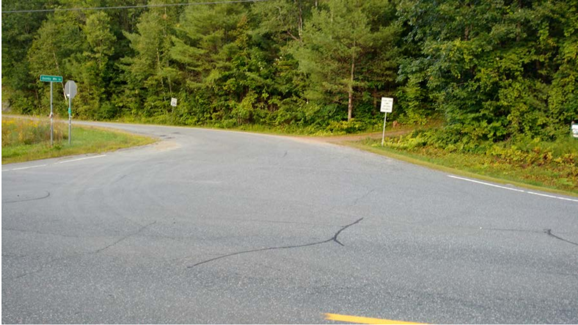
Quimby Mountain Road: Photo taken 8/31/2017 at station 0+00.
