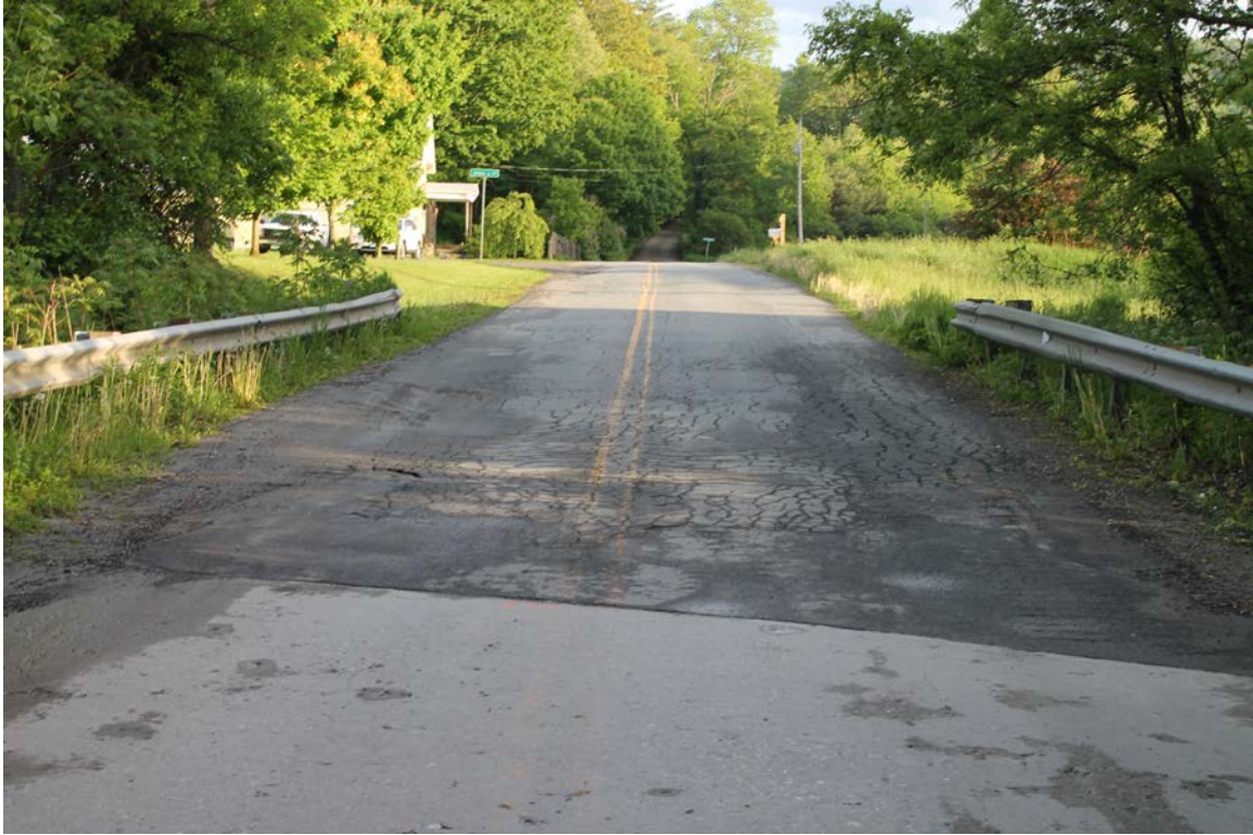
Broad Brook Road: Photo taken 5/31/2017 at station 10+00.
