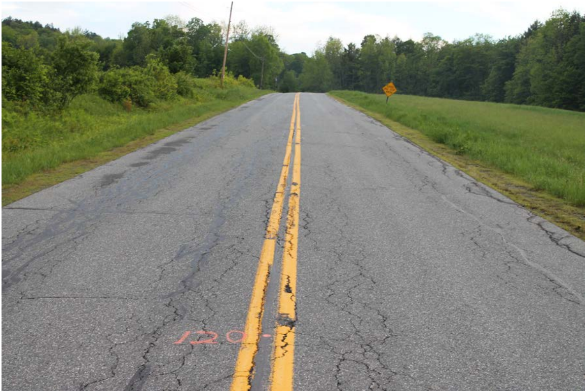
Howe Hill Road: Photo taken 5/31/2017 at station 120+00.
