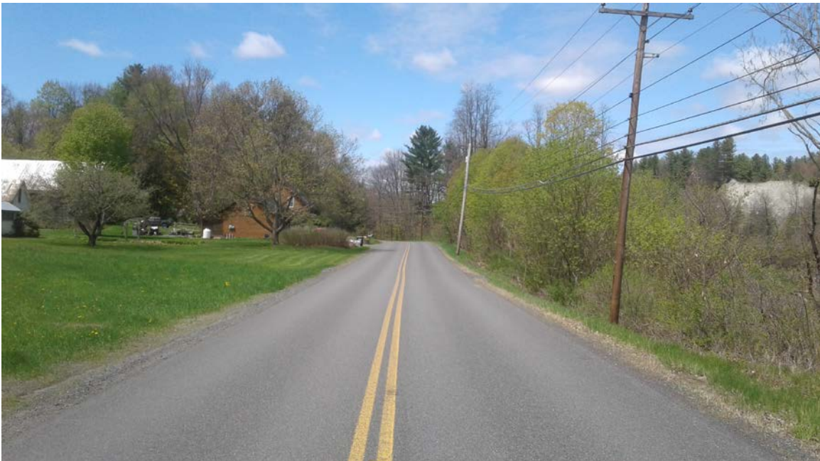
River Road: Photo taken 5/11/2017 at station 90+00.
