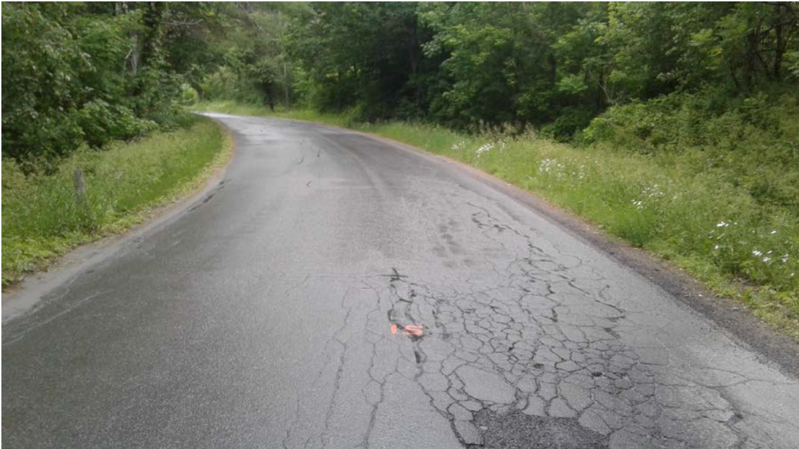
Fay Brook Road: Photo taken 6/29/2017 at station 15+00.
