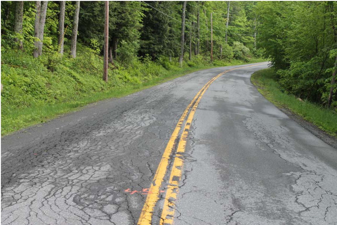
Howe Hill Road: Photo taken 5/31/2017 at station 45+00
