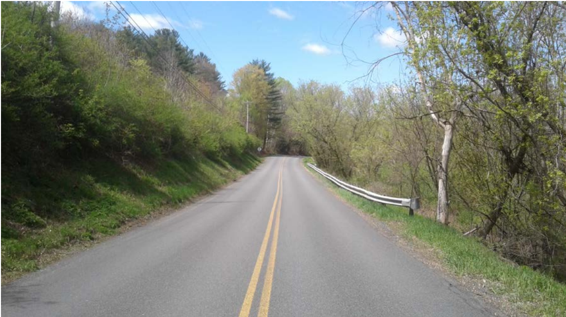
River Road: Photo taken 5/11/2017 at station 80+00.
