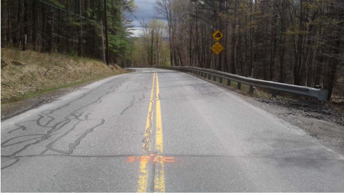
Rte #132: Photo taken 5/3/2017 at station 212+50.
