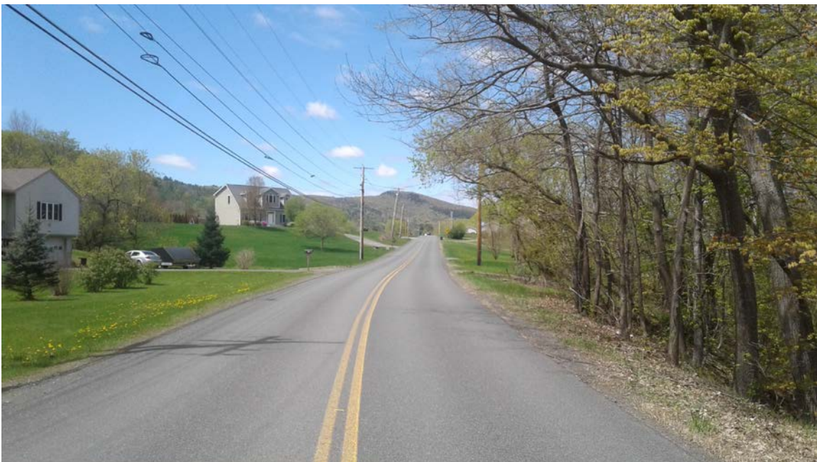
River Road: Photo taken 5/11/2017 at station 100+00.
