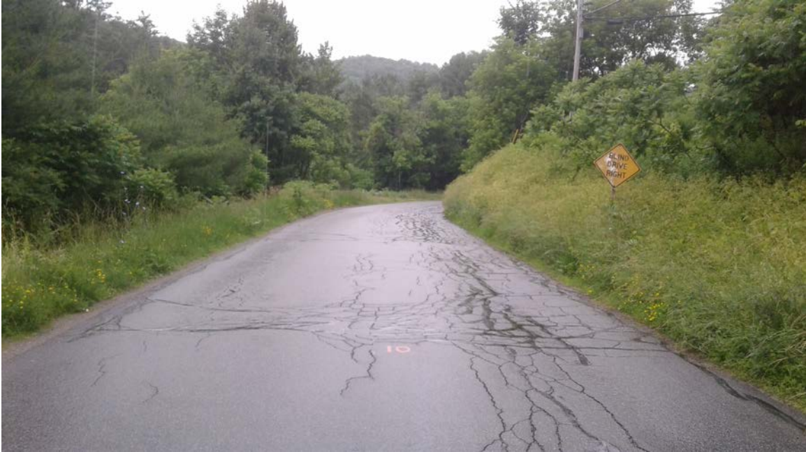
Fay Brook Road: Photo taken 6/29/2017 at station 10+00.
