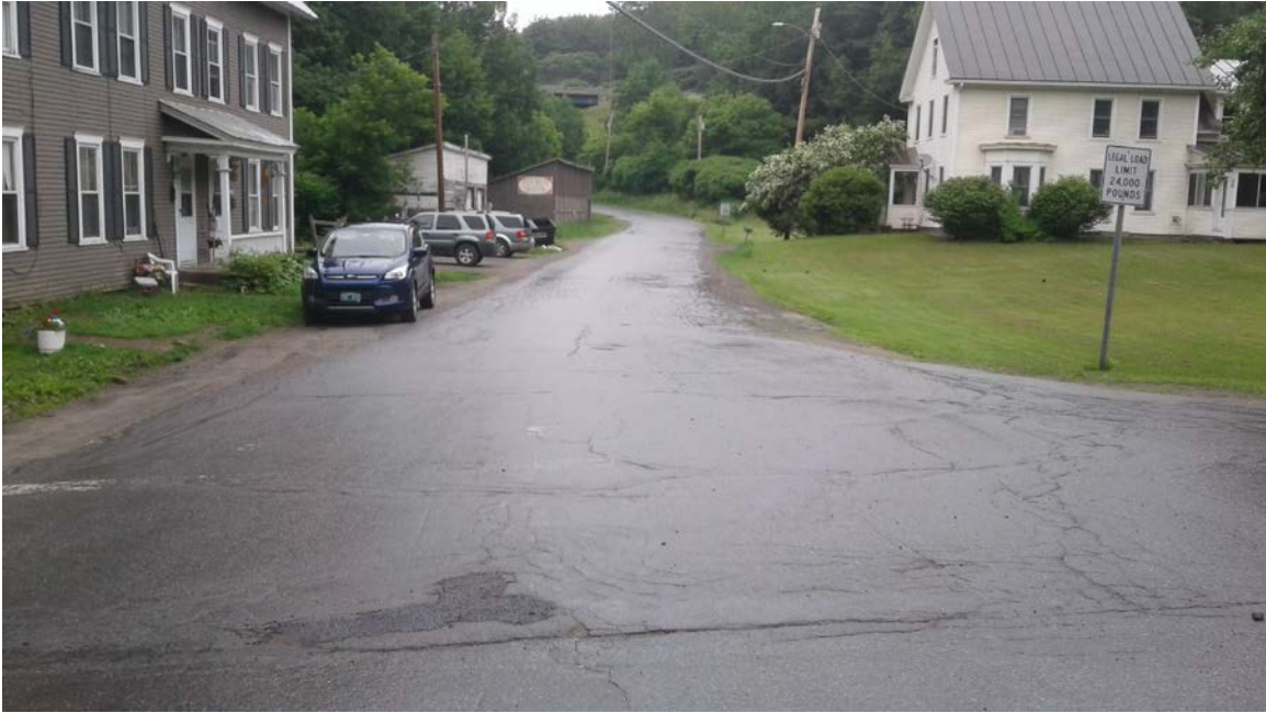
Fay Brook Road: Photo taken 6/29/2017 at station 0+00.
