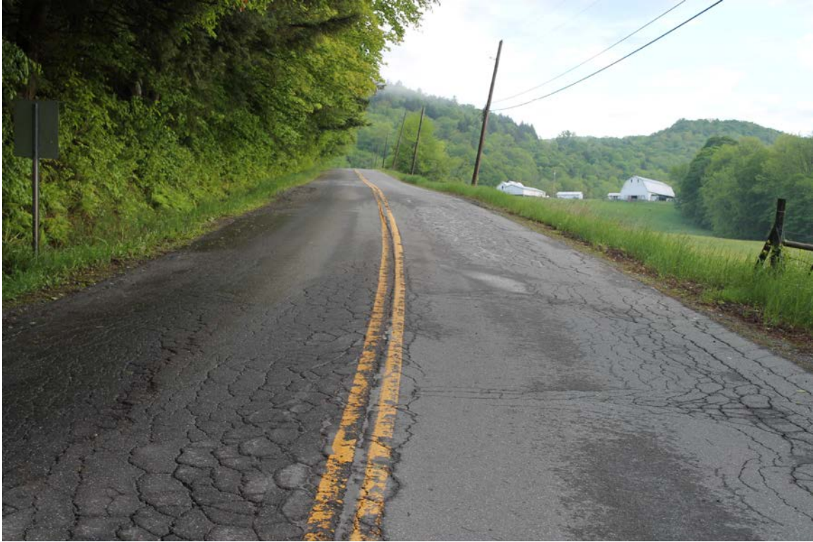
Howe Hill Road: Photo taken 5/31/2017 at station 20+00.
