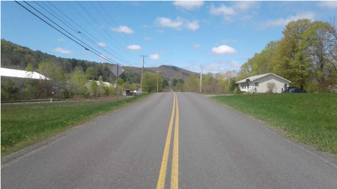
River Road: Photo taken 5/11/2017 at station 110+00.
