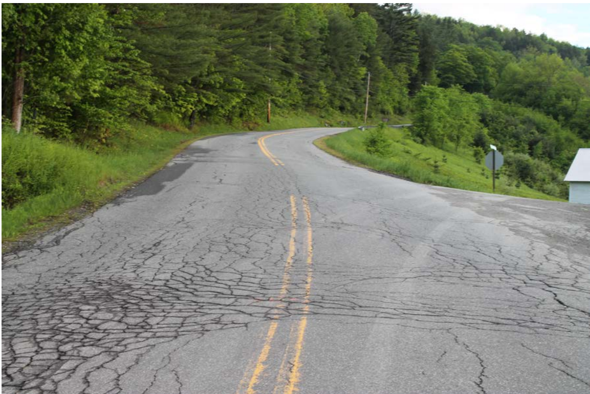
Howe Hill Road: Photo taken 5/31/2017 at station 35+00.
