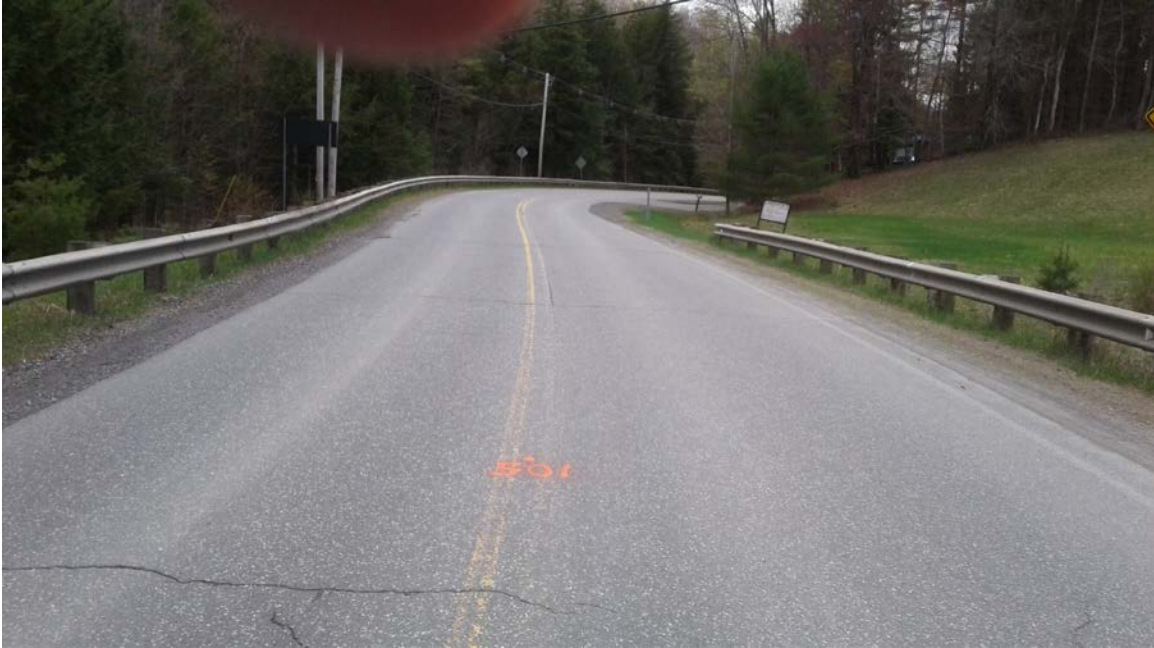
Rte #132: Photo taken 5/3/2017 at station 105+00.
