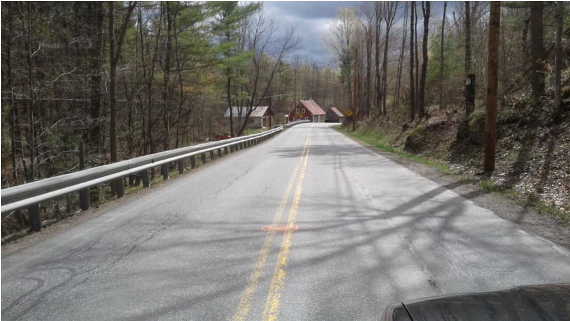
Rte #132: Photo taken 5/3/2017 at station 170+00.
