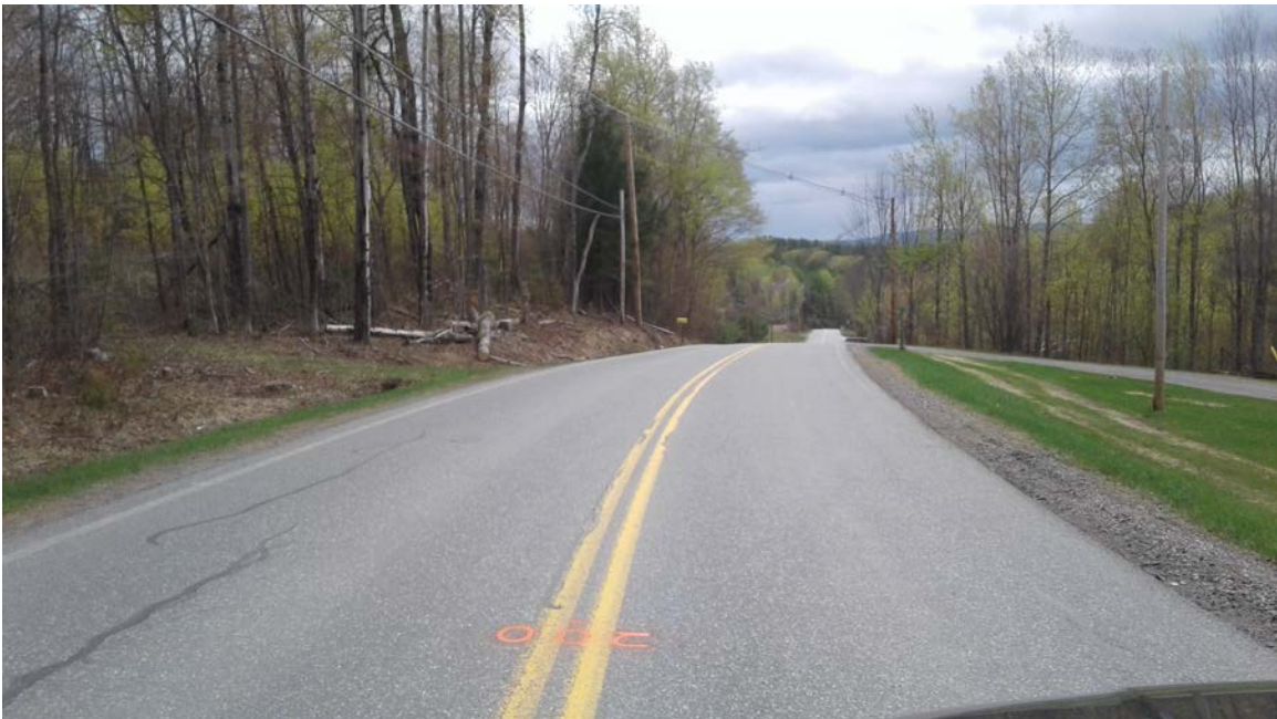
Rte #132: Photo taken 5/3/2017 at station 200+00.
