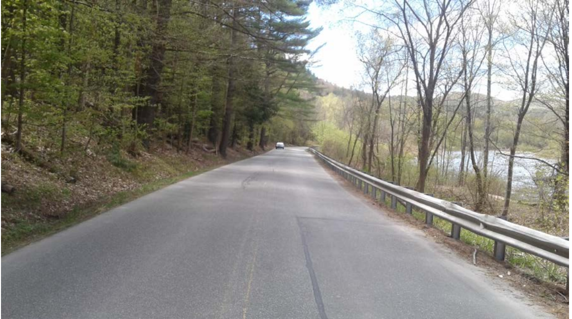
River Road: Photo taken 5/11/2017 at station 10+00.
