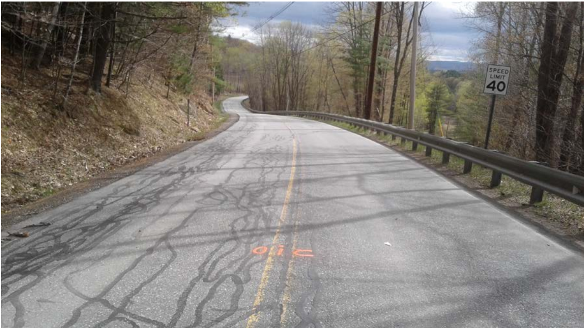
Rte #132: Photo taken 5/3/2017 at station 210+00.
