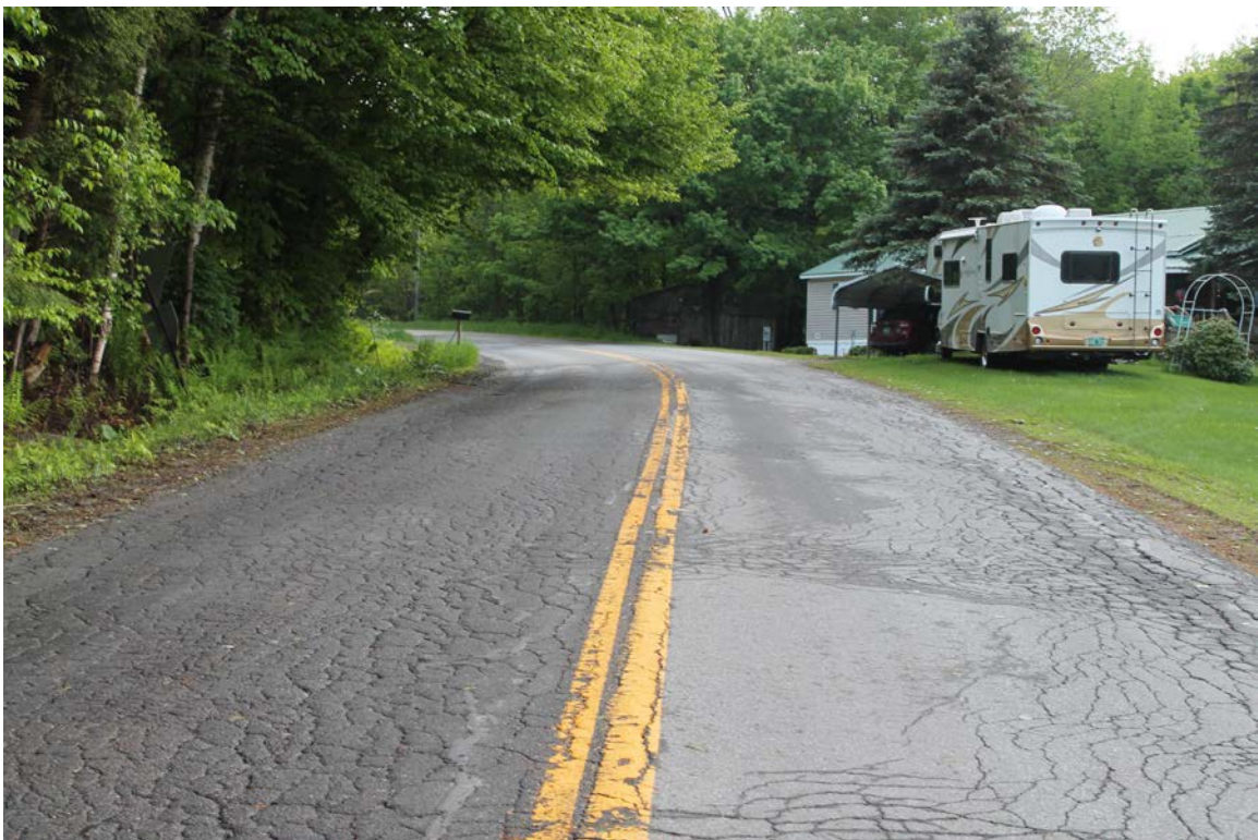
Howe Hill Road: Photo taken 5/31/2017 at station 5+00.
