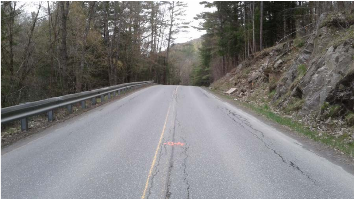
Rte #132: Photo taken 5/3/2017 at station 40+00.
