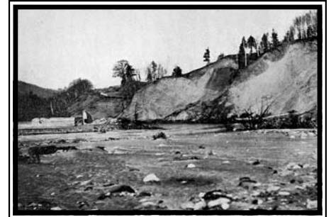
Huge washout at Sharon Dam
